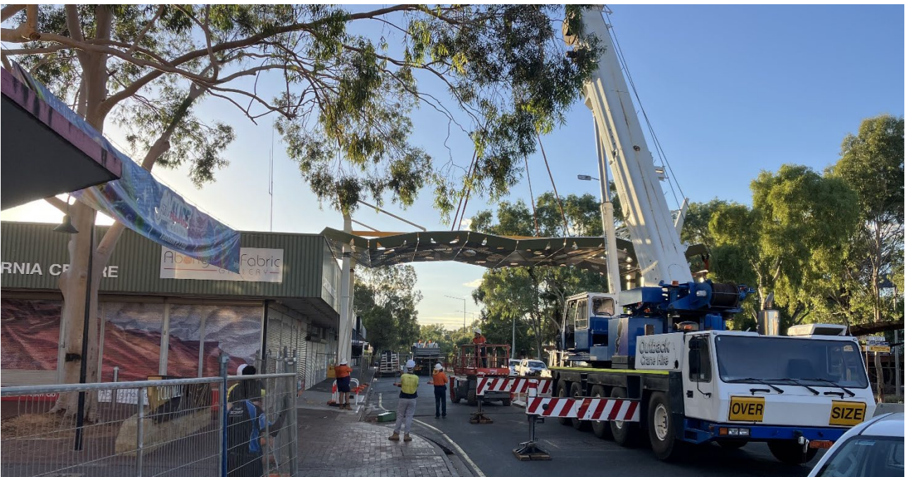
Alice Springs CBD - construct shade structures, landscaping, roadworks and associated works
