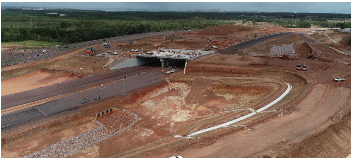
Tiger Brennan Drive - design and construct overpass at Berrimah Road intersection. Photos courtesy of Sitzler
