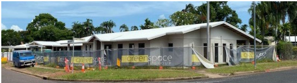
Wagaman and Wanguri - specialist disability accommodation - 2 dwellings Image courtesy of Carpentaria Disability Services
