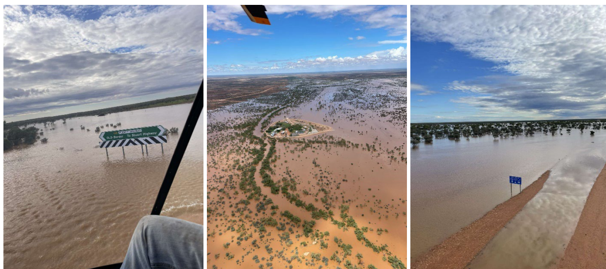
Flood impacted Plenty Highway - pavement repairs various sections ch 297 - 497 km
