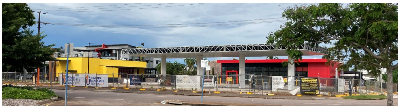
Stuart Park - 34 Stuart Highway - service station and food premises-fast food outlet
