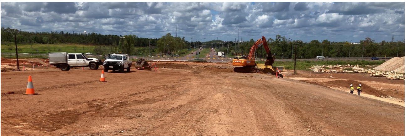
Tiger Brennan Drive - design and construct overpass at Berrimah Road Intersection
