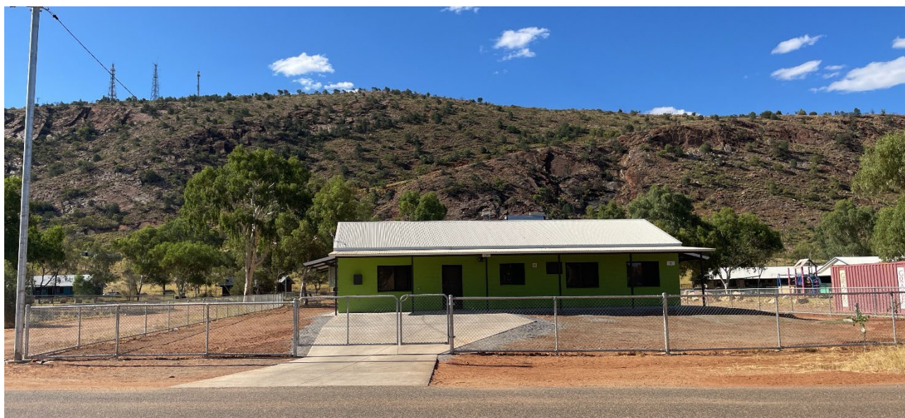
Karnte, Larapinta Valley, Little Sisters, Morris Soak and Trucking Yards Town Camps - demolish and construct housing (4 by packages - A, B, C and D)
