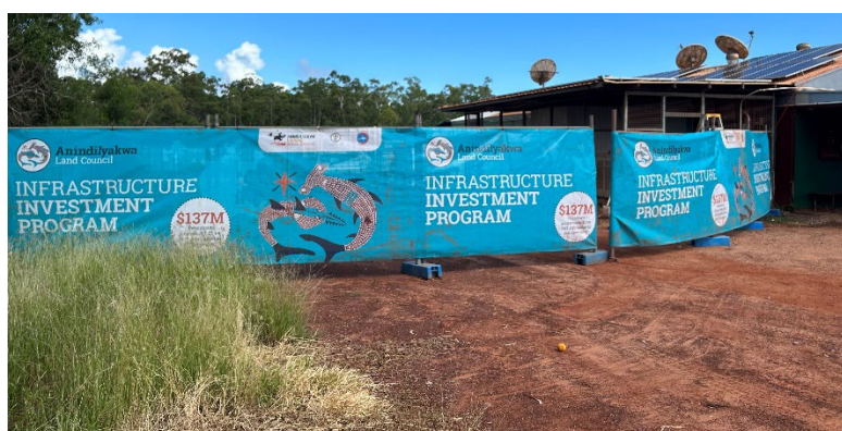
Outback Store upgrades
