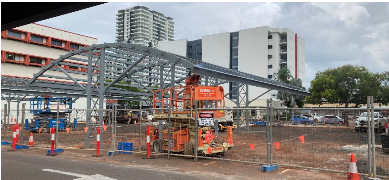
Darwin CBD - Woolworths carpark expansion and new access via Searcy Street
