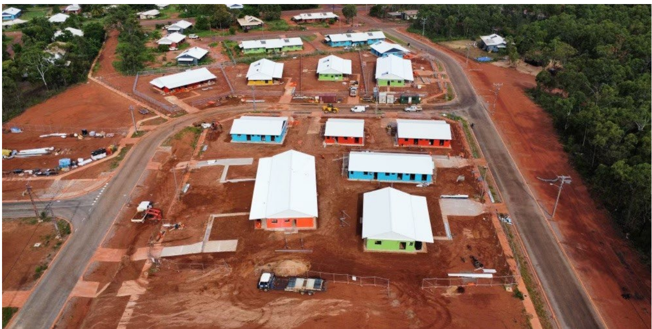
Yirrkala - construct 13 homes
