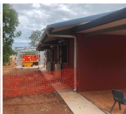
Cyclone shelter upgrades
