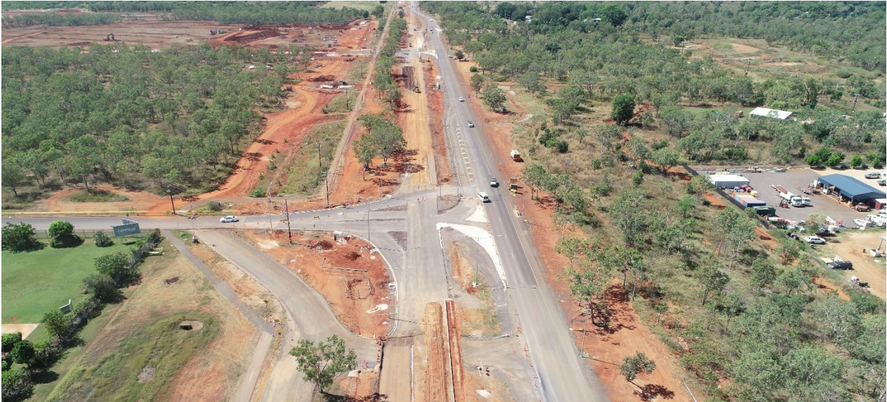
Stuart Highway duplication between Cyprus Street and Uralla Road ch 317.90 - 319.012 km
