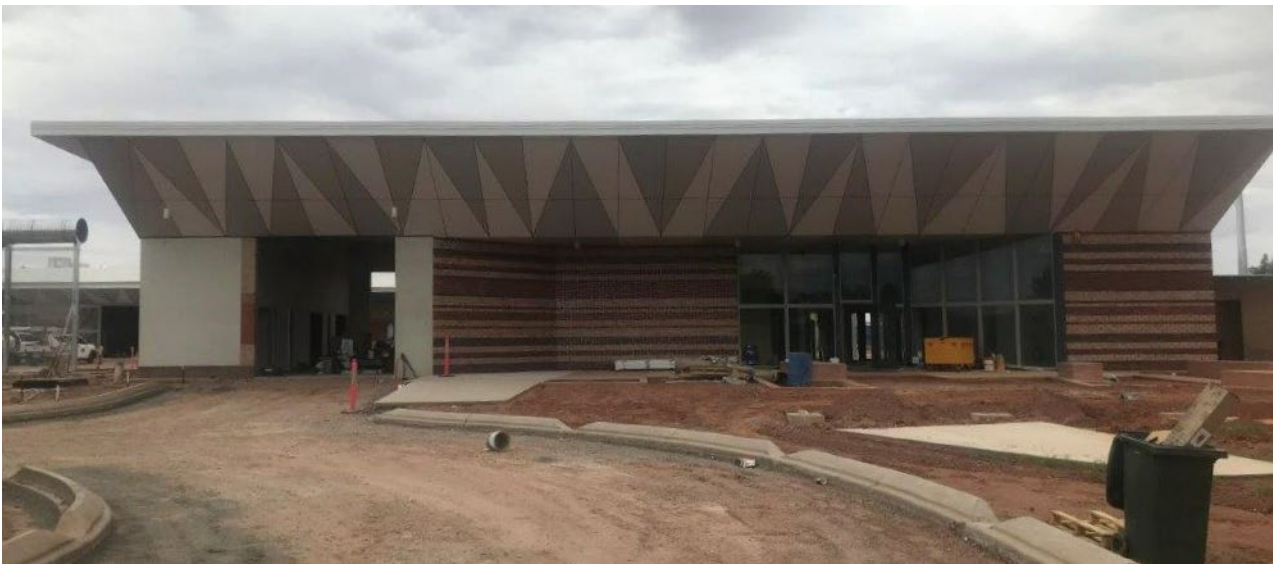
Alice Springs - youth detention centre - redevelopment
