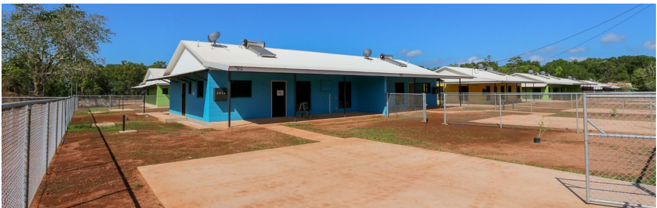
Pirlangimpi - construct 18 homes
