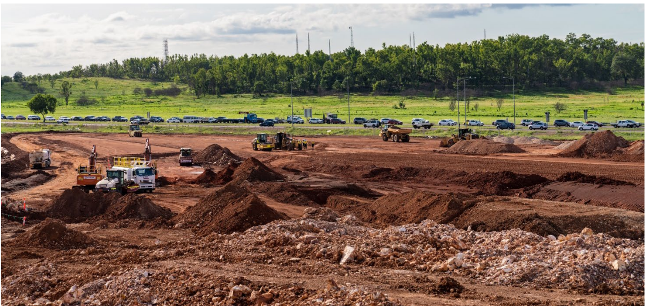
Tiger Brennan Drive - design and construct overpass at Berrimah Road intersection
