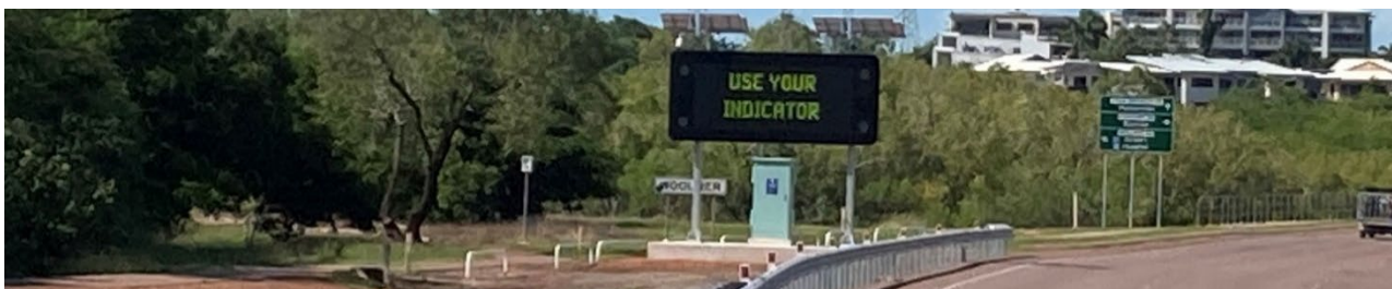
Various Highways - design, supply and install (28) variable message signs
