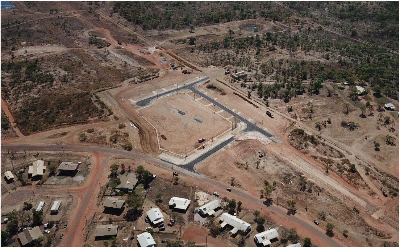
Gunbalanya (Oenpelli) - subdivision civil works and services construction
