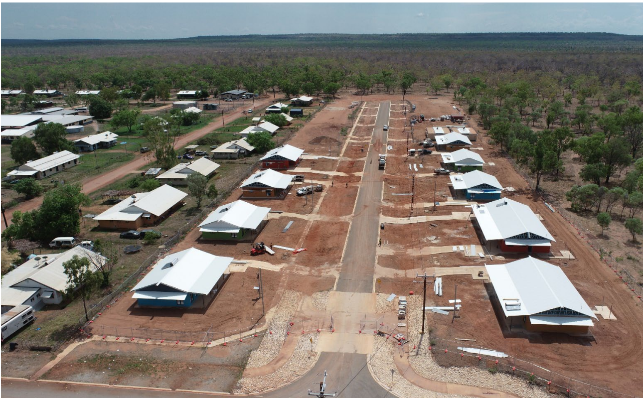
Beswick - construction works for housing infrastructure
