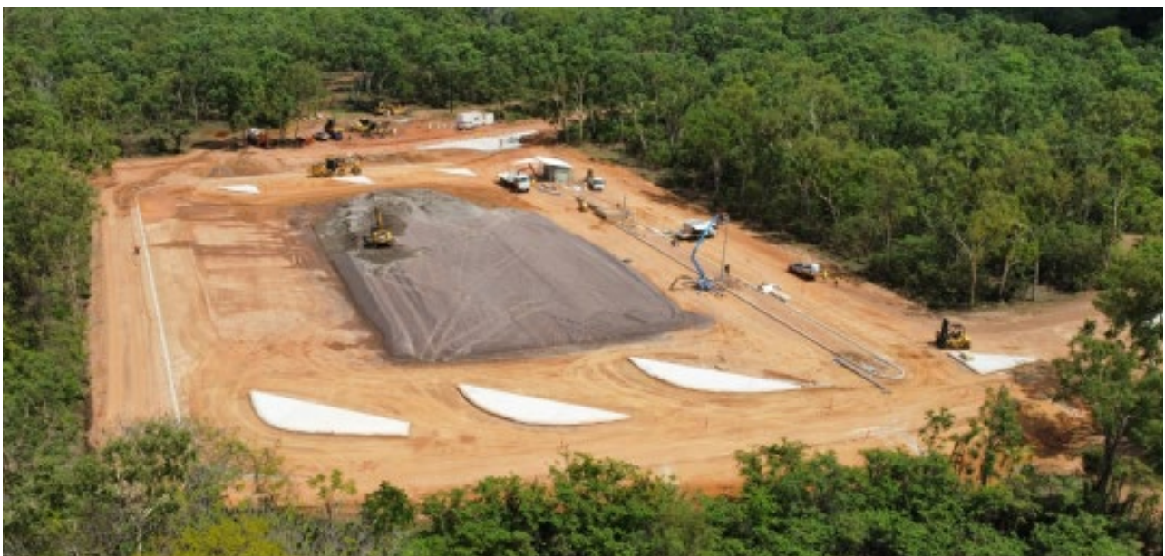
Daly River - construct new boat ramp, carpark and toilet facilities
