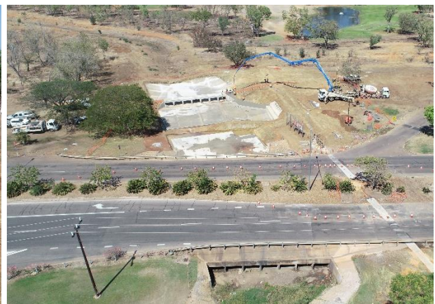
Katherine Township - flood mitigation levee (Northern Section)
