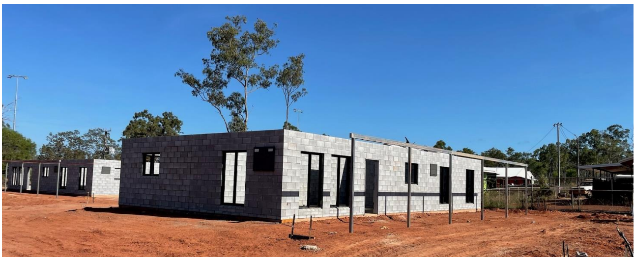
Gapuwiyak - construct, refurbish and upgrade NTG housing infrastructure
