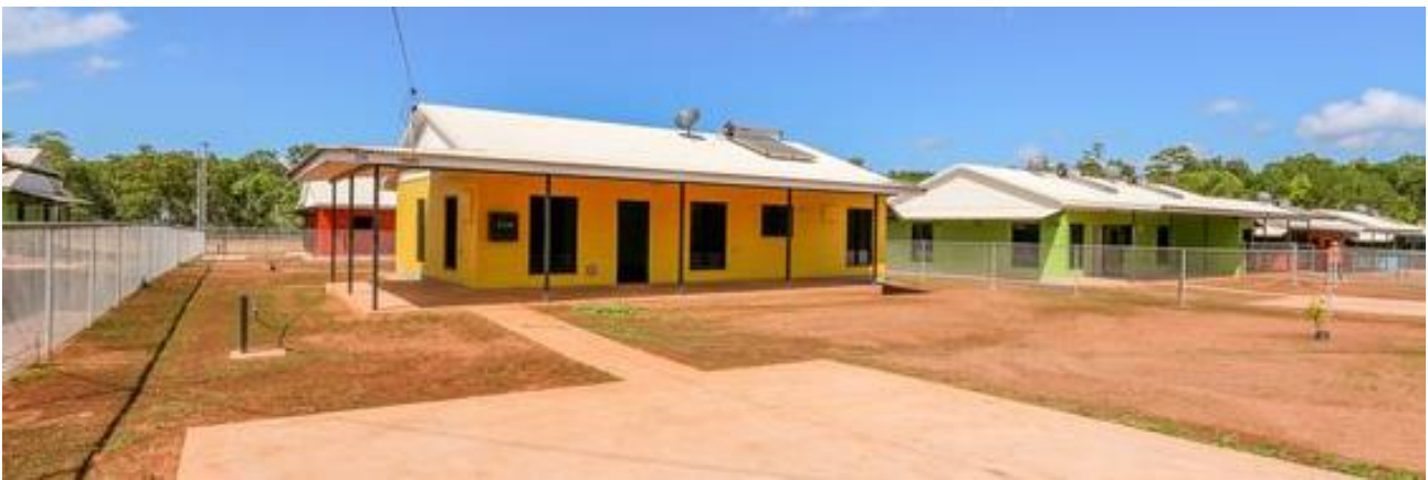
Pirlangimpi - construct 18 homes
