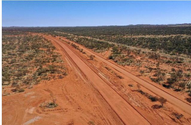
Tanami Road - upgrade and sealing between chainage 271.81 - 421.0 km
