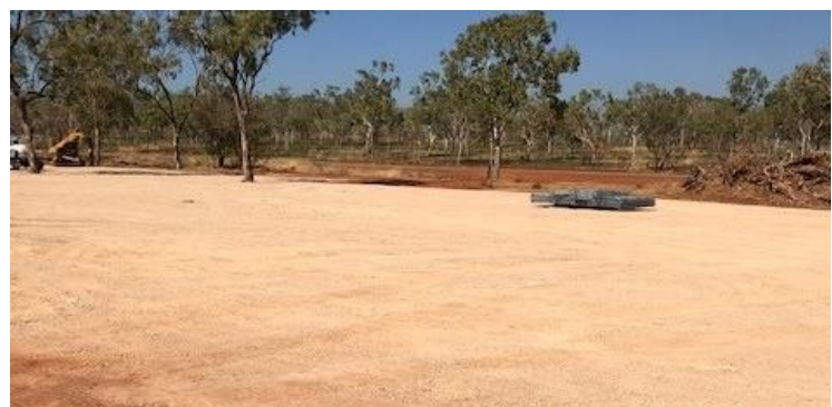
Binjari - relocate buildings from Bottom Camp to Top Camp and refurbish. Images courtesy of Binjari Community Aboriginal Corporation
