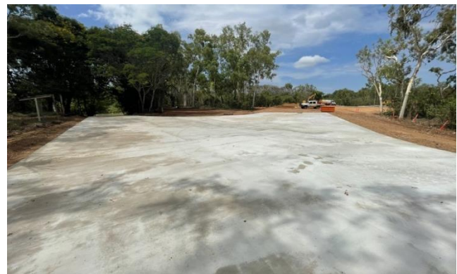
Daly River - construct new boat ramp carpark and toilet facilities
