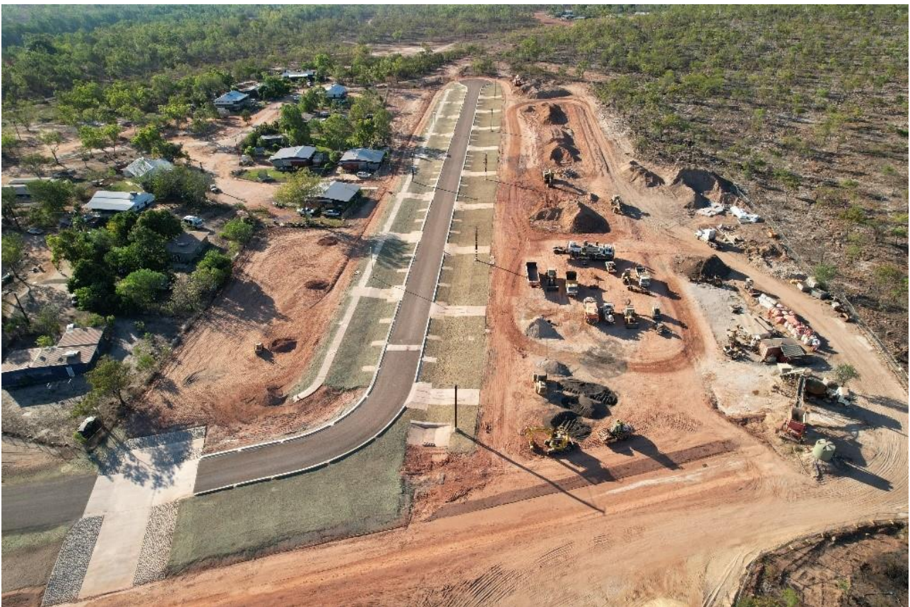
Borroloola - Garawa 2 - subdivision civil works and services construction
