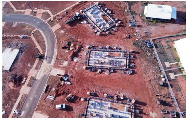
Yirrkala - construct 13 homes
