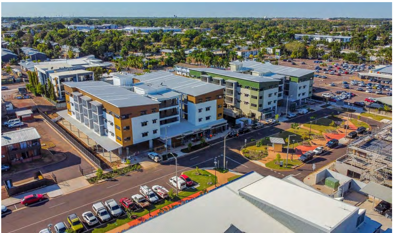
Nightcliff - John Stokes Square redevelopment - residential precinct construction
