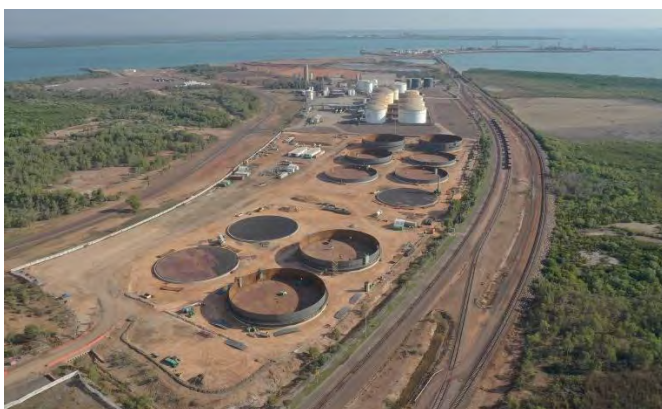
East Arm - Bulk Liquids Area – Crowley Project Caymus - construct U.S Defence jet fuel storage facility
