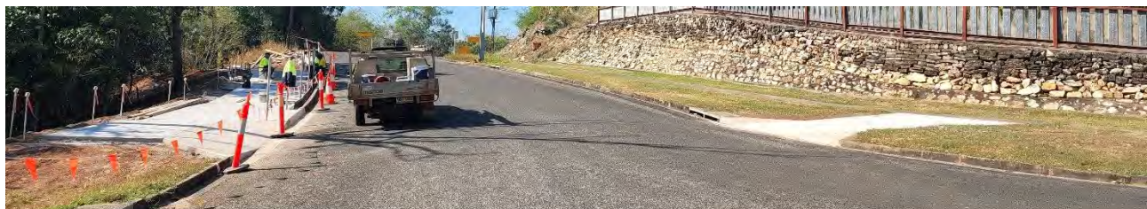
Stuart Park to Woolner - construct shared path and ramp
