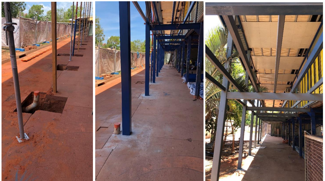
Photos: Galiwinku - Shepherdson College - replace verandas and associated works
