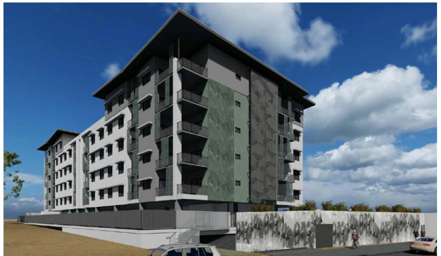
IMAGE COURTESY OF WHITTAKER STREET DEVELOPMENTS
