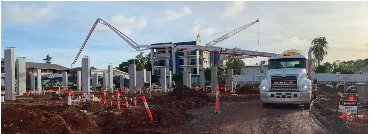
Photos: Nightcliff - John Stokes Square redevelopment - residential precinct construction
