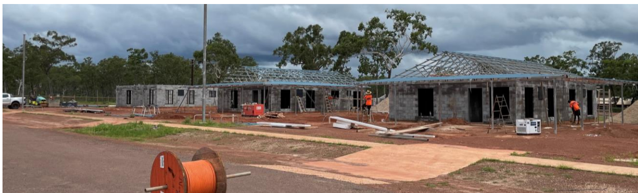
Construction photos: Gapuwiyak construct 10 dwellings
