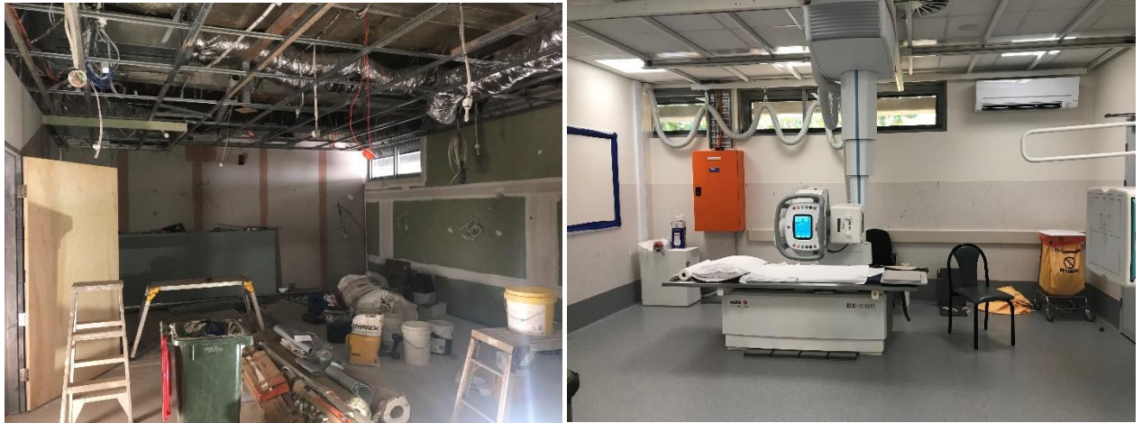
Photos: Gove District Hospital - upgrade imaging department
