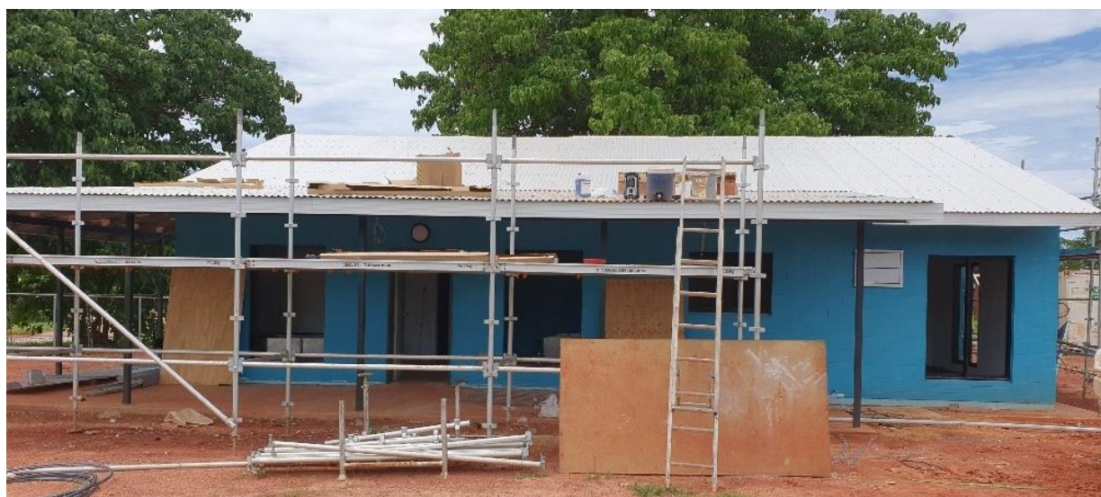
Construction photos: Maningrida - HomeBuild NT - construct 12 dwellings
