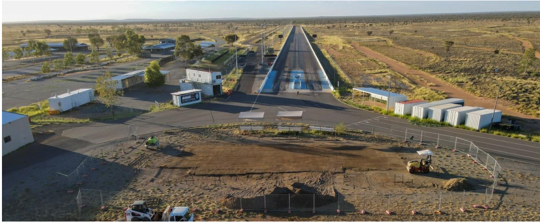
Construction photo: Central Australian Drag Racing Association - construct race control tower
