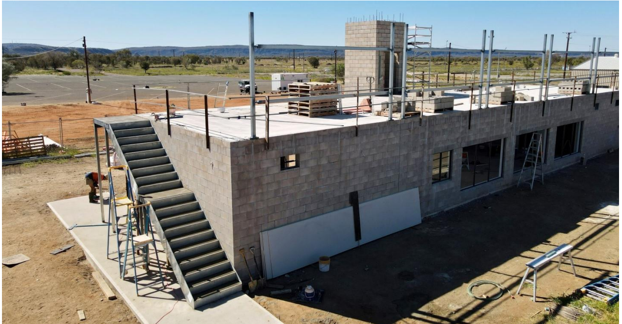
Construction photo: Central Australian Drag Racing Association - construct race control tower
