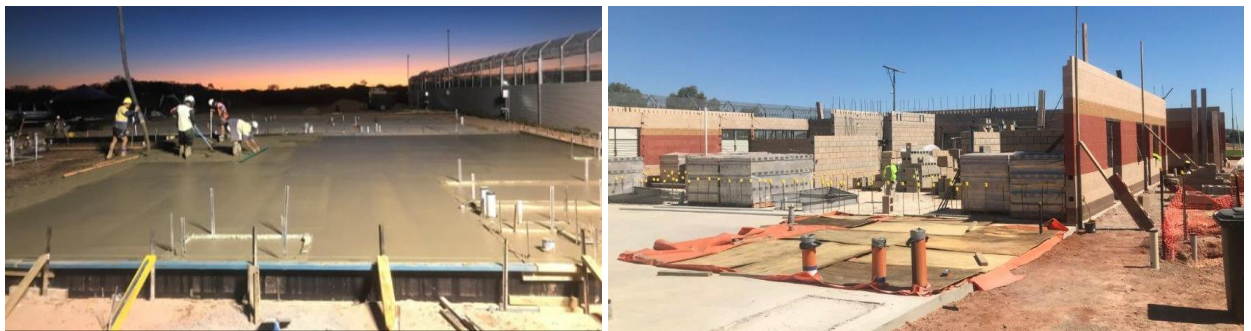
Construction photos: Alice Springs - youth detention centre - redevelopment
