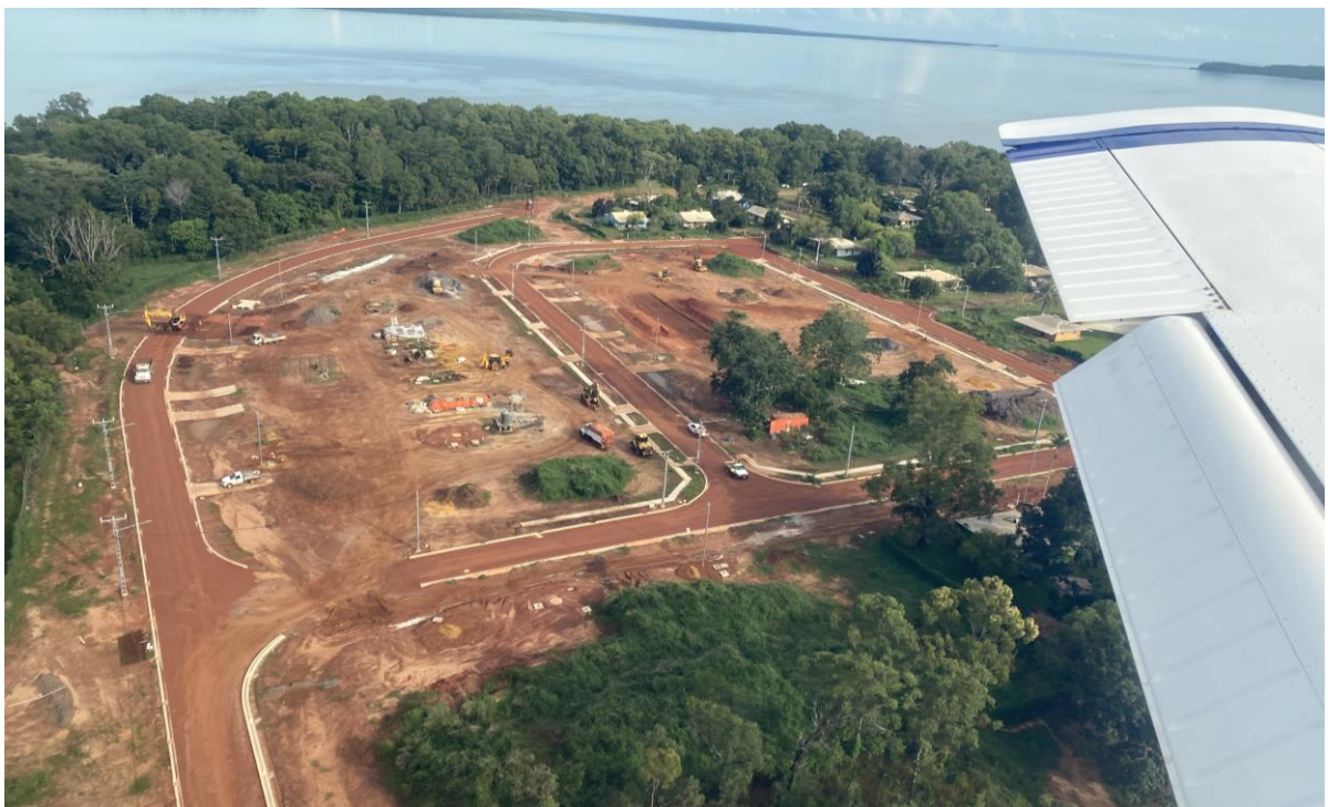
Construction photo: Pirlangimpi - subdivision civil works and services construction
