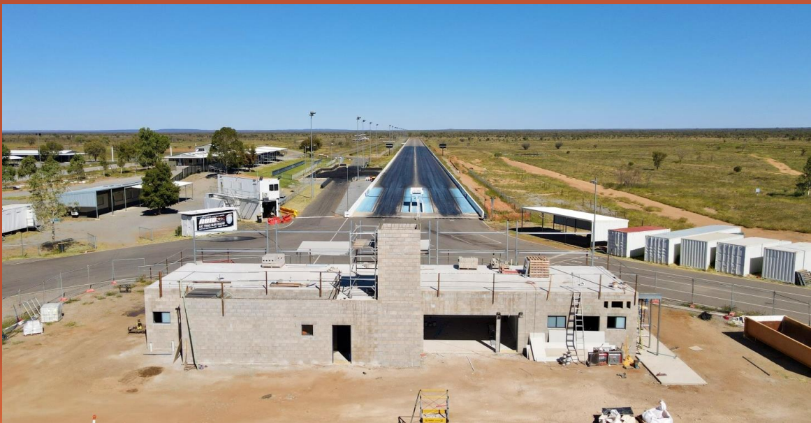
Alice Springs – Central Australian Drag Racing Association - construct race control tower
