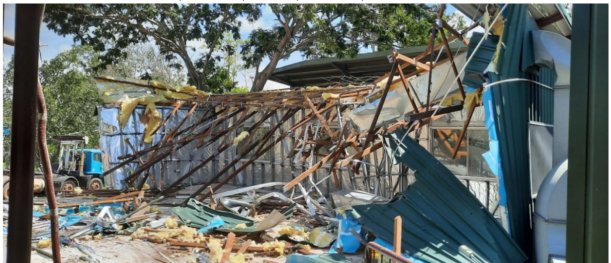
Demolition photo: Leanyer Primary School - replace classroom block
