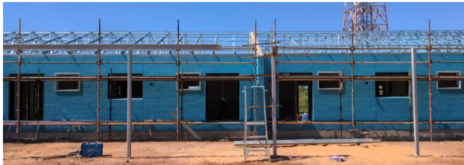
Construction photos: Yarralin - NPRH Program - construct 6 new dwellings
