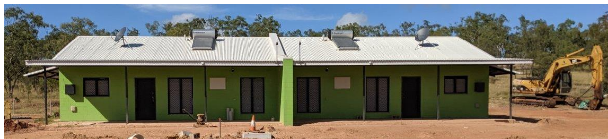
Construction photos: Borroloola - Garawa 1 Town Camp - duplex
