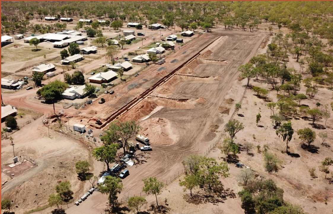
Beswick - subdivision civil works and services
