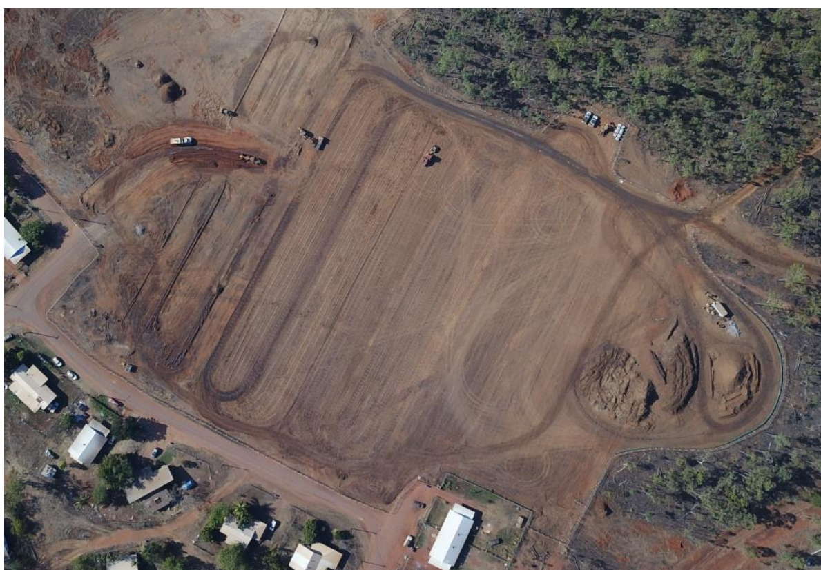
Construction photo: Ramingining - subdivision civil works and services construction
