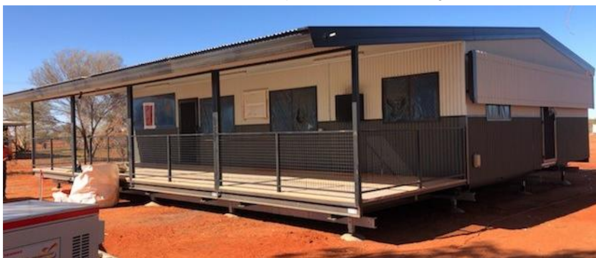
Photo: Finke - NPRH NT - pre-fabs - construct 4 dwellings
