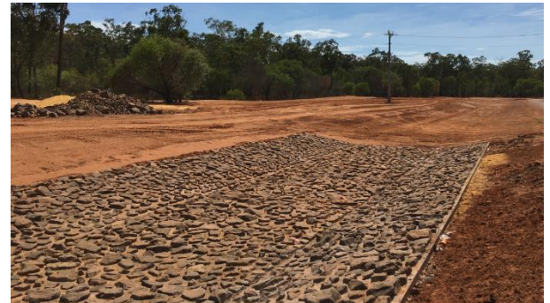
Construction photos: Maningrida subdivision - drainage remediation works
