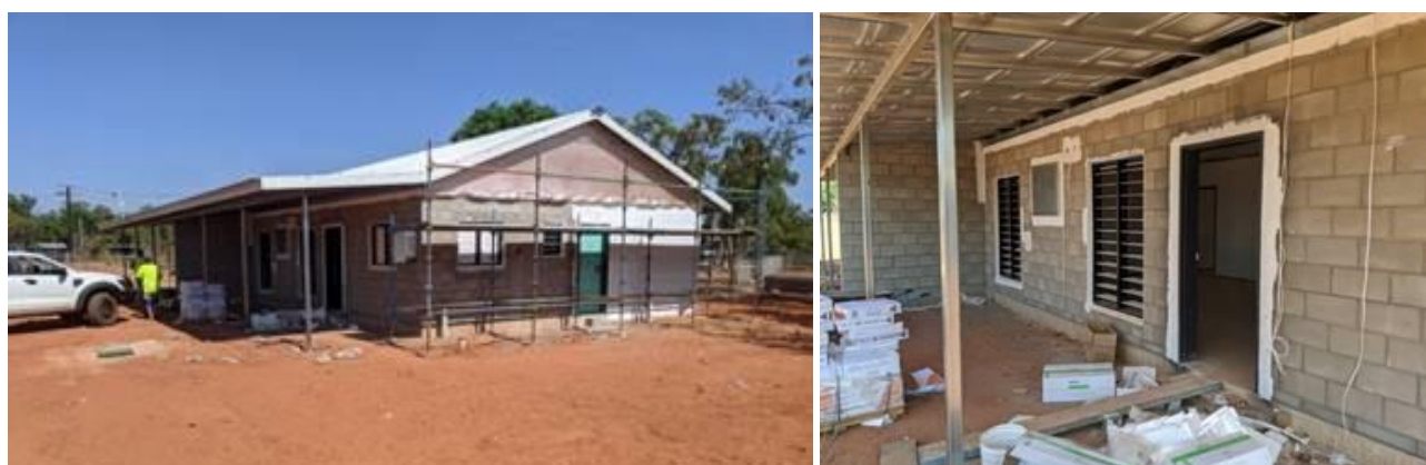
Photos: Borroloola - Mara Town Camp - construct 4 dwellings
