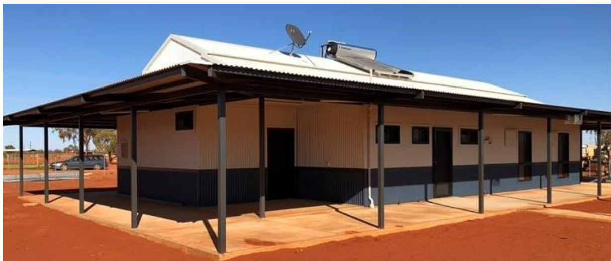
Photo: Kintore - NPRH NT - construct 5 dwellings
