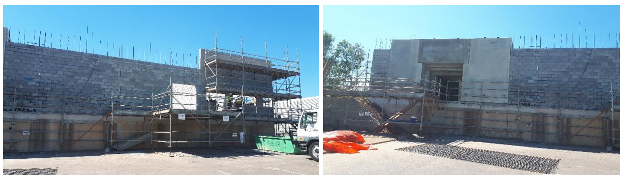
Construction photos: Royal Darwin Hospital - chemotherapy chair expansion and cyclotron facility
