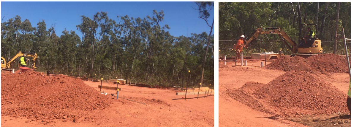
Construction photos: Yirrkala (lots 236 & 237) - HomeBuild NT - construct 2 by 3 bedroom duplexes
