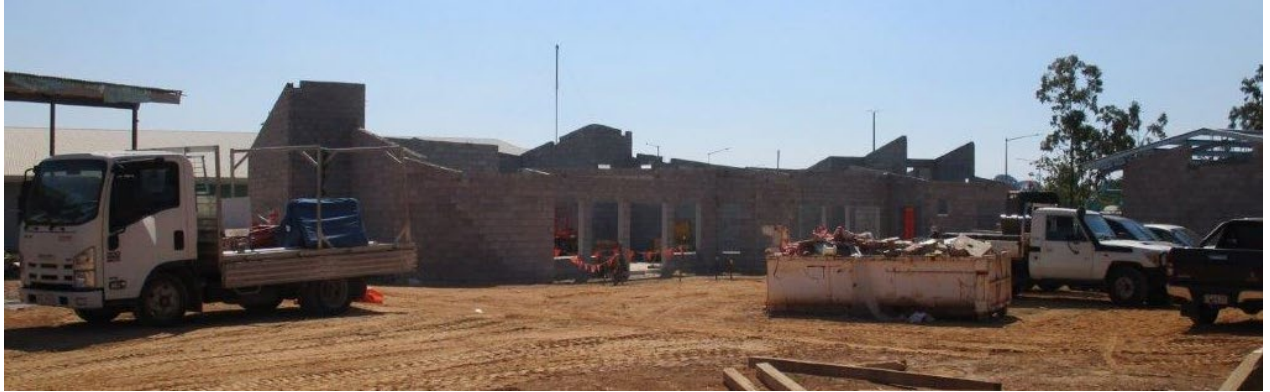
Construction photos: Zuccoli Primary School - stage 2 of the government school
