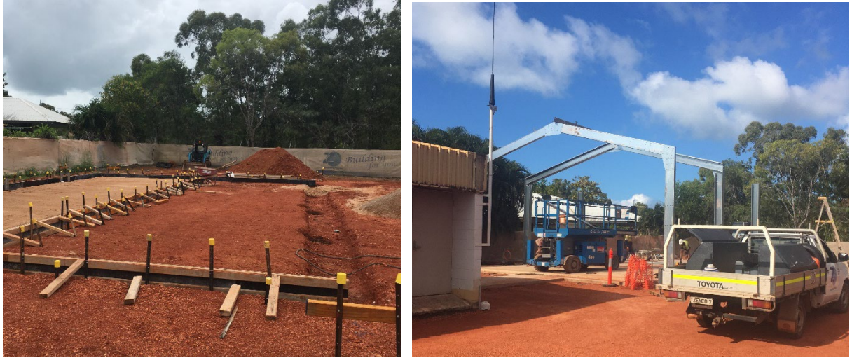
Construction photos: Nhulunbuy - design and construct new NTES shed
