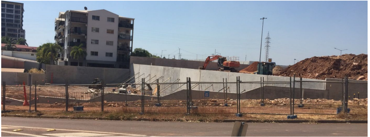
Construction photo: Darwin CBD - 33 Daly Street - site establishment project
