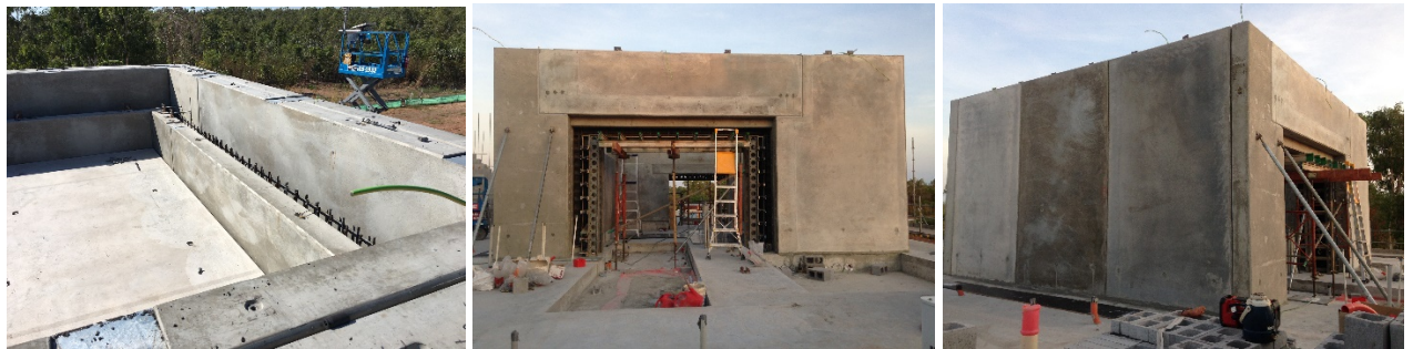
Construction photos: Royal Darwin Hospital - chemotherapy chair expansion and cyclotron facility
