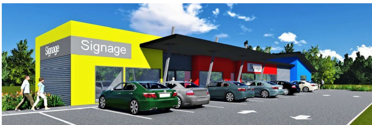
Concept: Durack - Packard Avenue - medical clinic and childcare centre in single storey building
