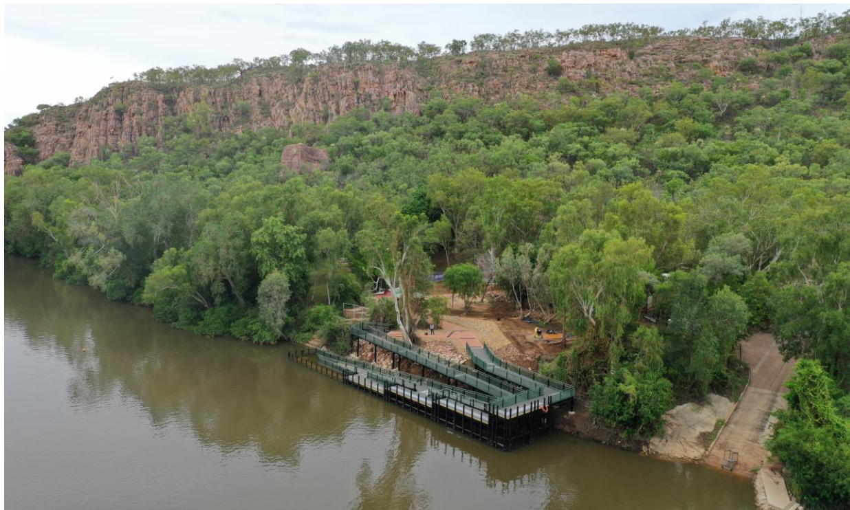
Construction photo: Nitmiluk National Park - construct new tour boat jetty
