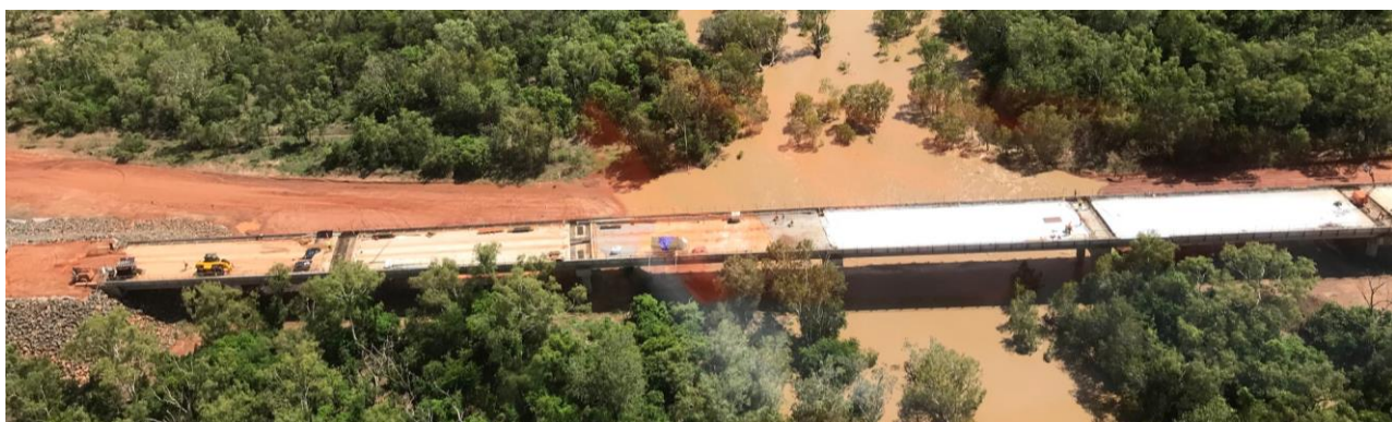
Construction photo: Keep River Plains Road - upgrade chainage 0 - 26.7 km
