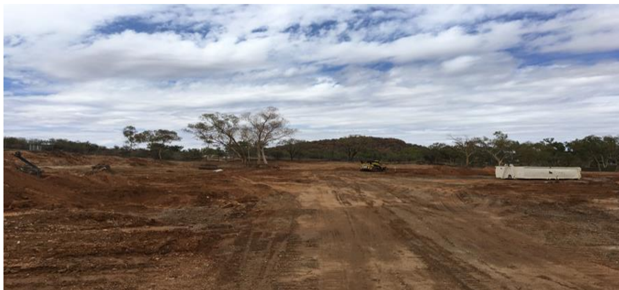
Construction photo: Anzac Hill School- demolition works
