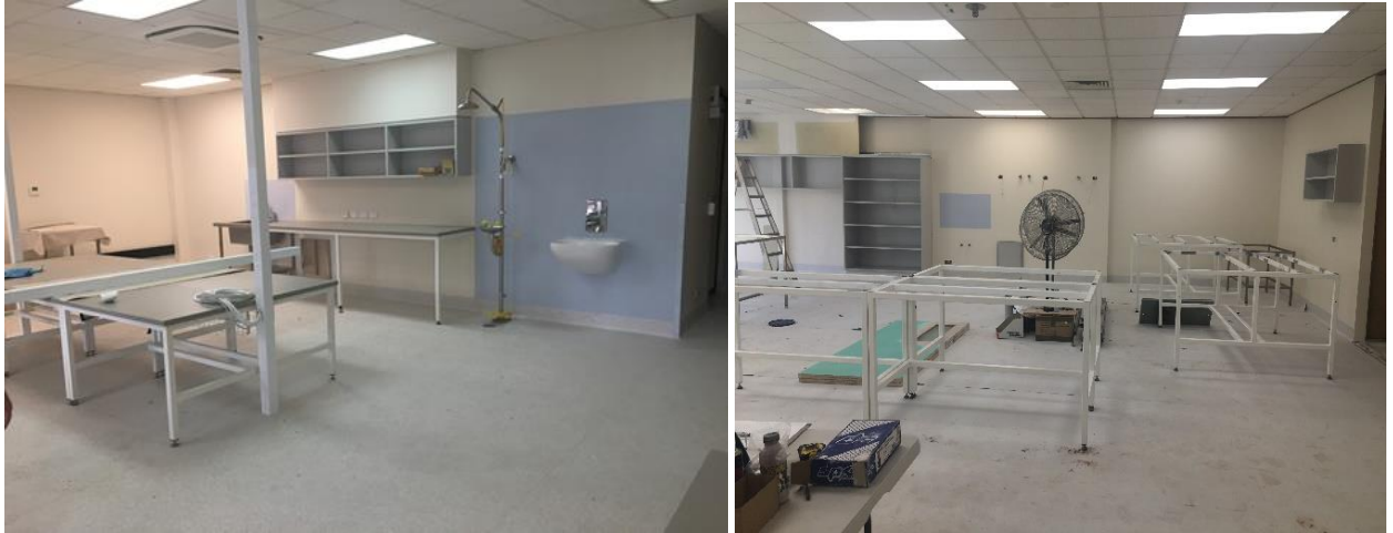
Construction photos: Alice Springs Hospital – Liebig Building pathology fit out
