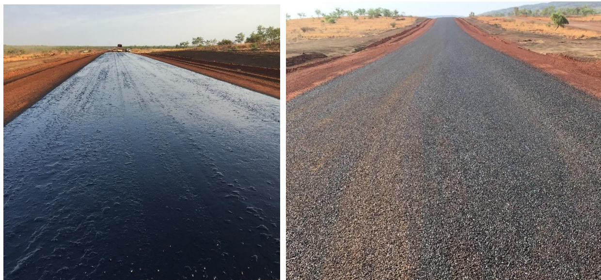
Construction photos: Tablelands Highway - strengthening and widening chainage 287 - 303 km
