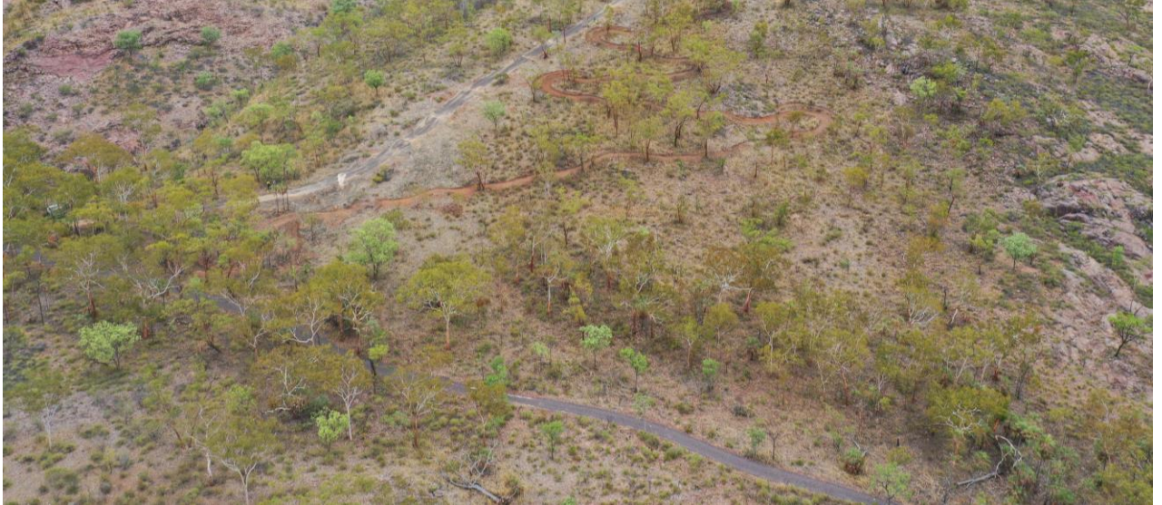
Construction photos: Nitmiluk National Park - Mountain bike trail construction
