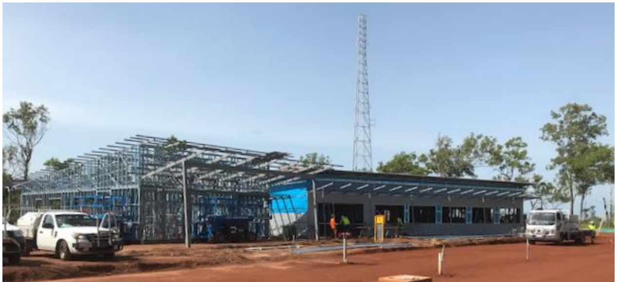
Construction photo: Acacia Hills - construct new Bushfires NT headquarters
