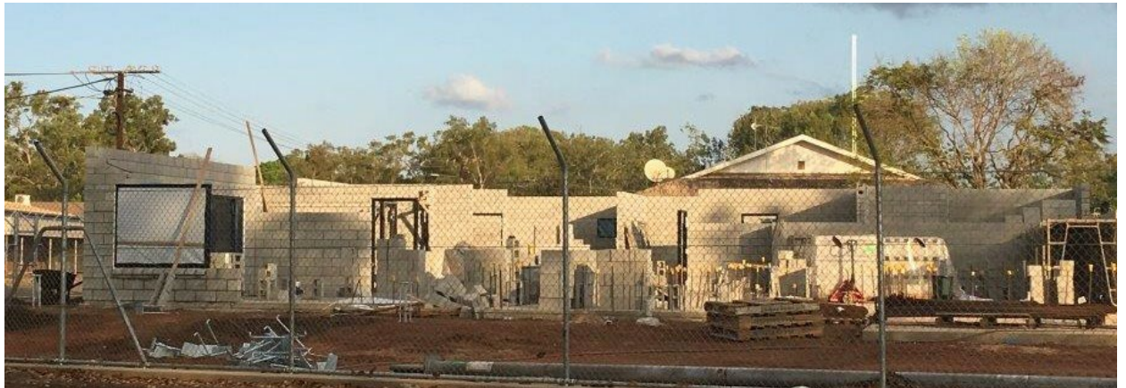
Construction photos: Angurugu - new permanent police post including multi-function area
