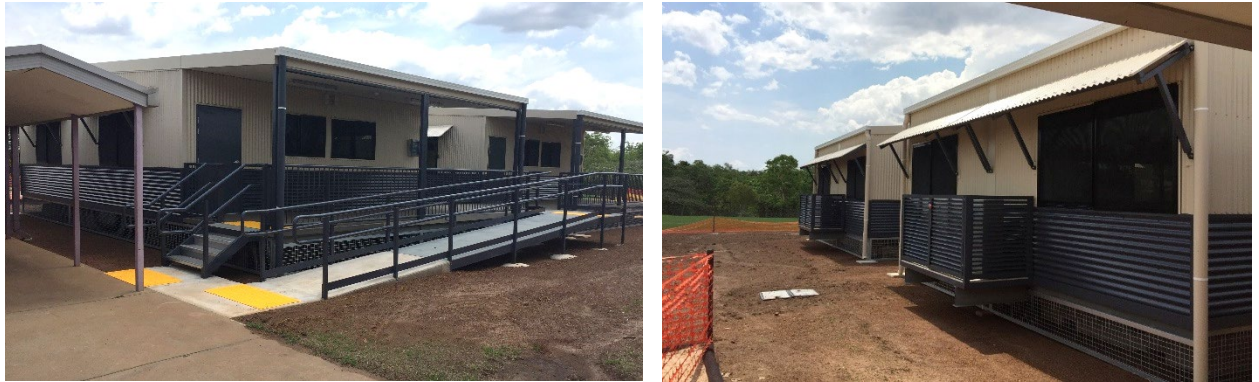
Construction photos: Girraween Primary School - new general learning area
