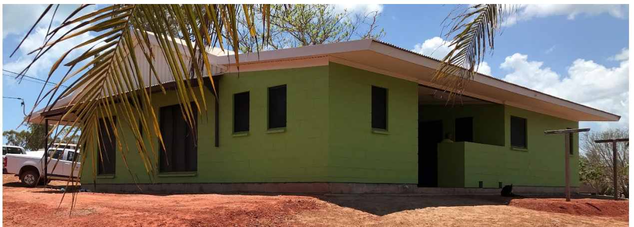
Construction photo: Galiwinku - construct 8 by 4 bedroom dwellings
