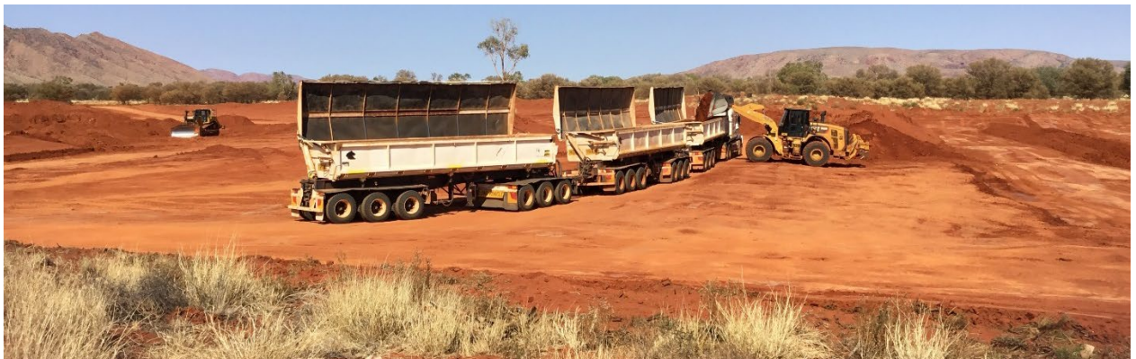
Construction photos: Tjukururu Road - upgrade between chainages 181 - 189 km
