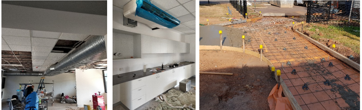
Construction photos: Henbury School - refurbish blocks E and F
