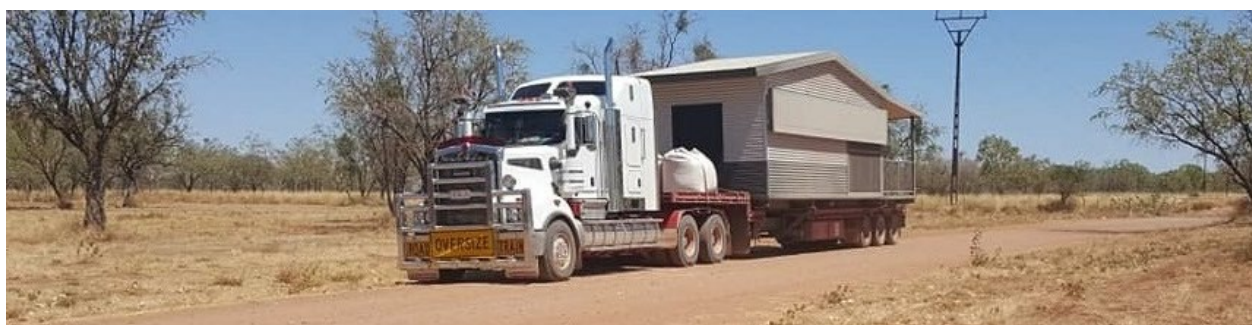
Transport photo: Yarralin - construct 5 prefabricated dwellings
