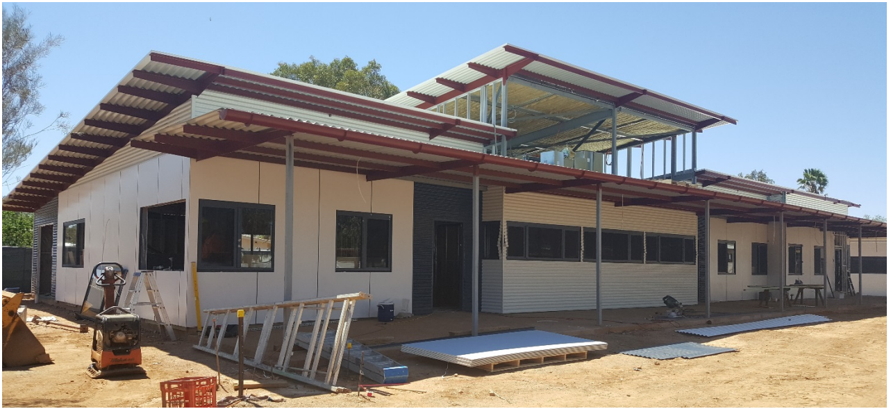
Construction photo: Acacia Hill School - upgrades
