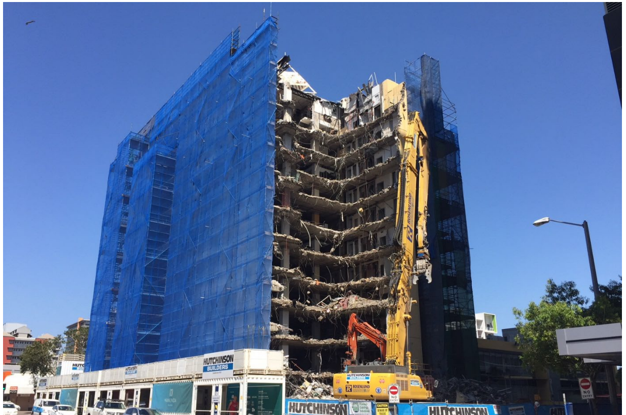
Demolition photo: Darwin CBD - 38 Cavenagh Street - demolition of 9 storey building
