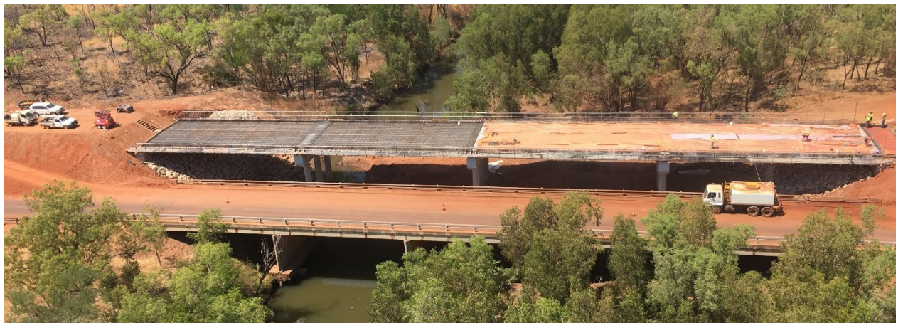
Construction photo: Victoria Highway - Little Horse and Big Horse Creek upgrade
