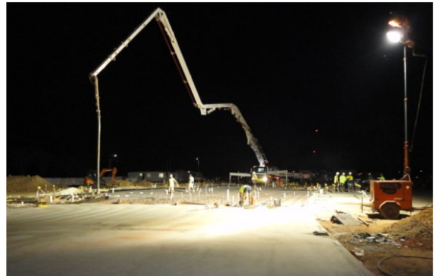
Construction photos: Katherine - new Fire Station
