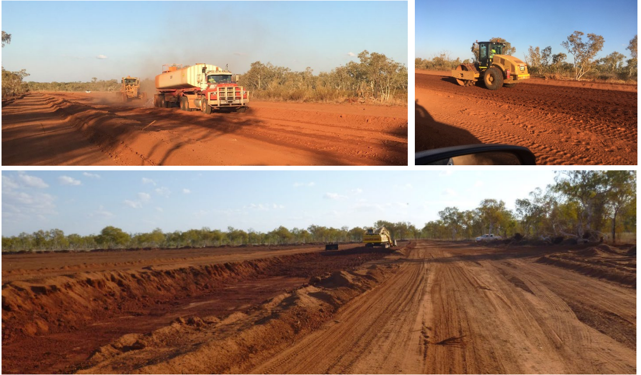
Construction photos: Buntine Highway - upgrades between chainage 372 - 387 km
