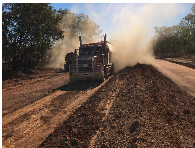
Construction photo: Stuart Highway - upgrade Cutta Cutta Caves intersection
