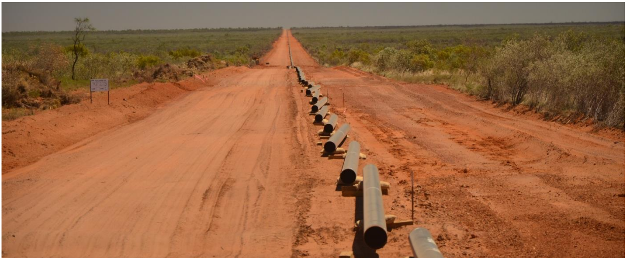
Construction photos: Northern Gas Pipeline - 622 kilometre pipeline
