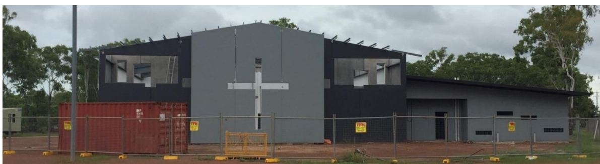
Construction photo: Howard Springs - 85 Whitewood Road - place of worship
