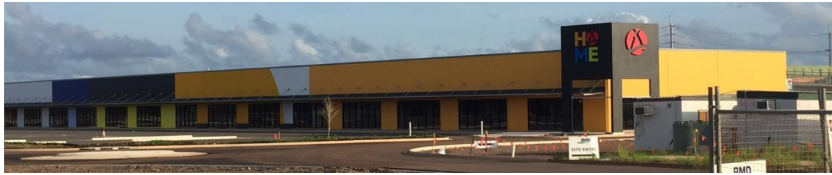
Construction photo: Palmerston - Gateway Shopping Centre - stage 3 - homemaker centre
