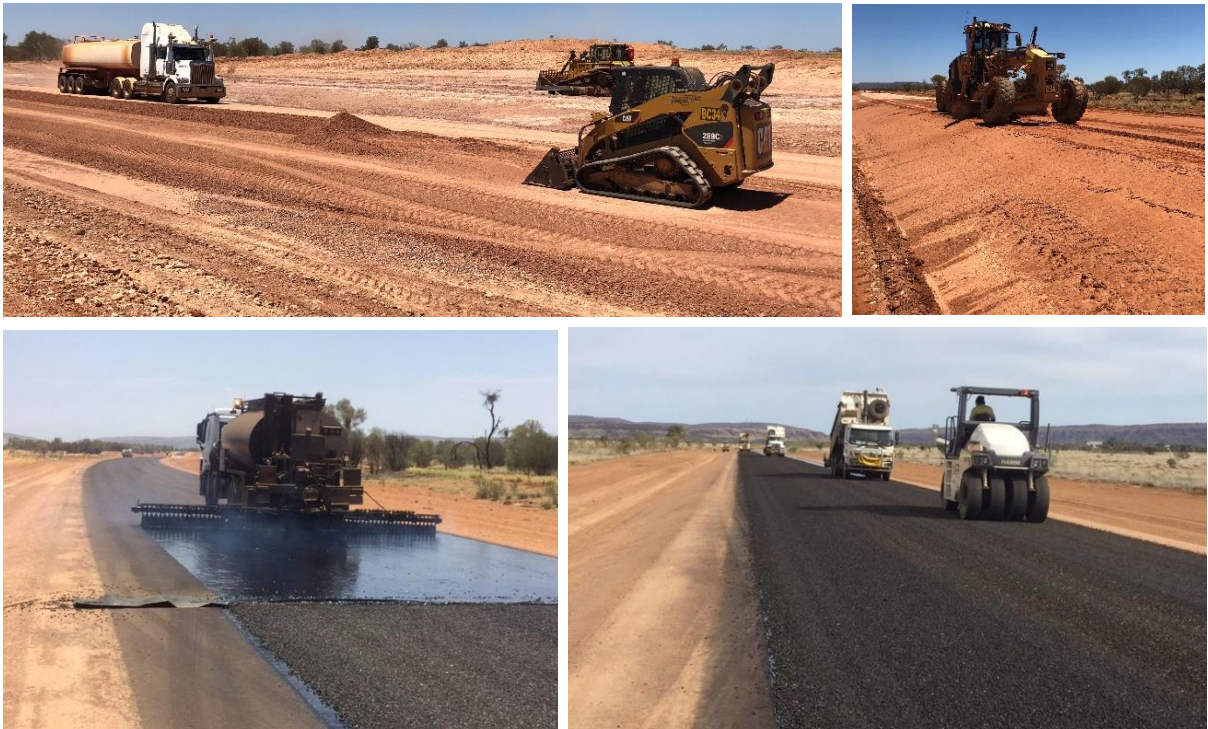
Construction photos: Maryvale Road - upgrade and seal
