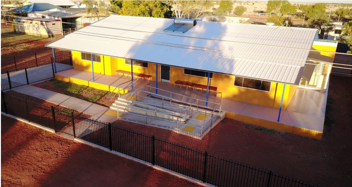
Construction photo: Alpurrurulam - new preschool
