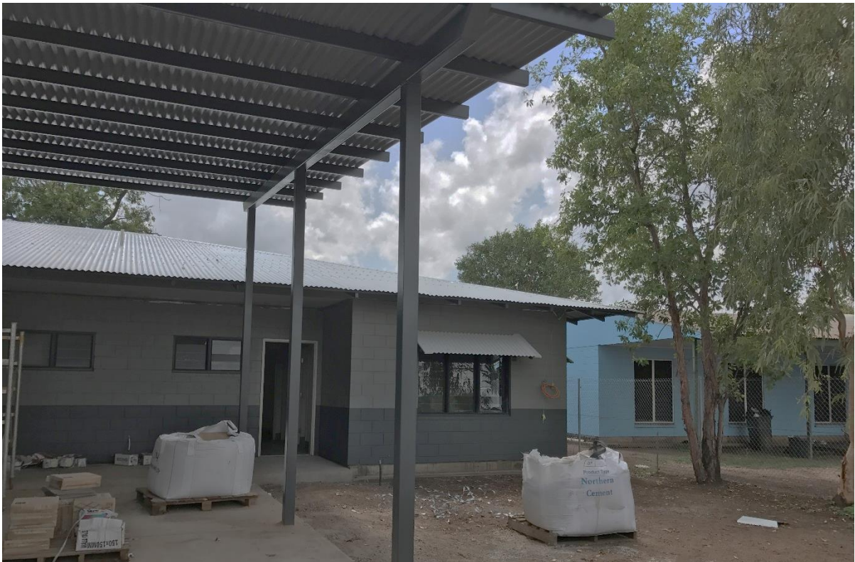
Construction photo: Gunbalanya (Oenpelli) - construct duplex
