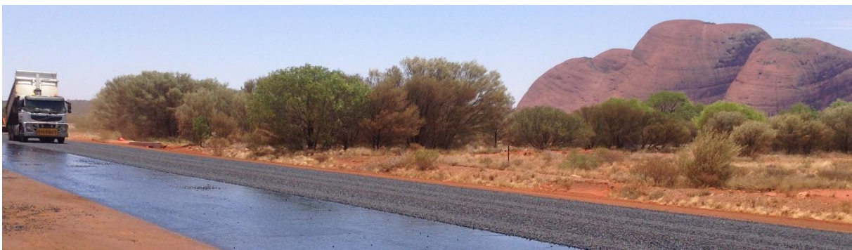
Construction photo: Tjukururu Road - chainage 0.8 - 8.8 km - upgrade and seal
