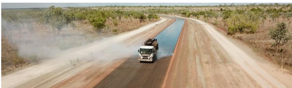
Construction photo: Roper Highway - road upgrade and seal from chainage 133.347 - 135.396 km
