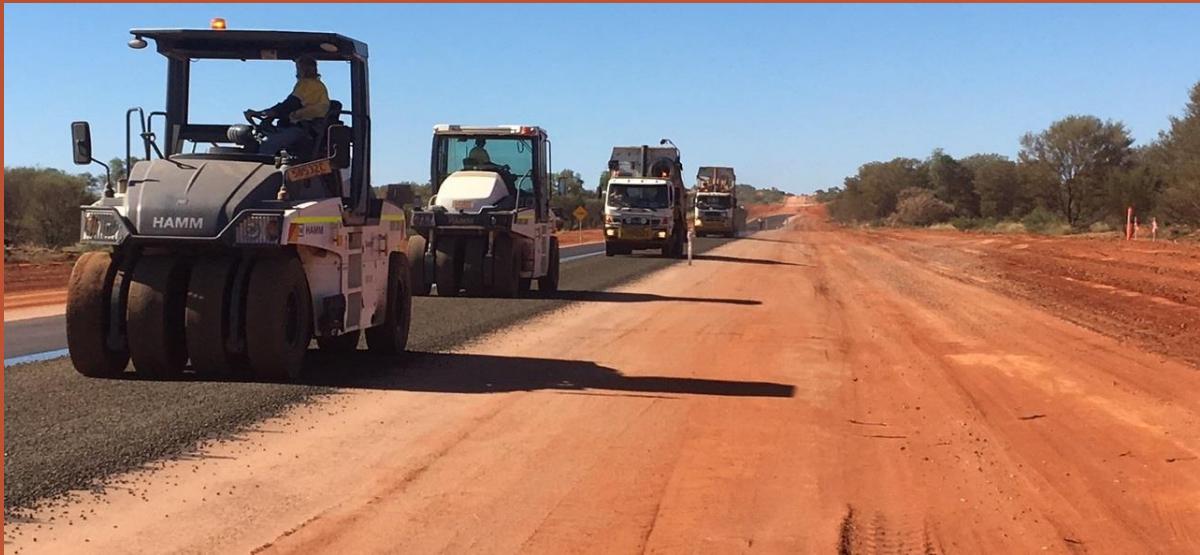
Maryvale Road - construct floodway at chainage 18.5 - 19.6 kilometres
