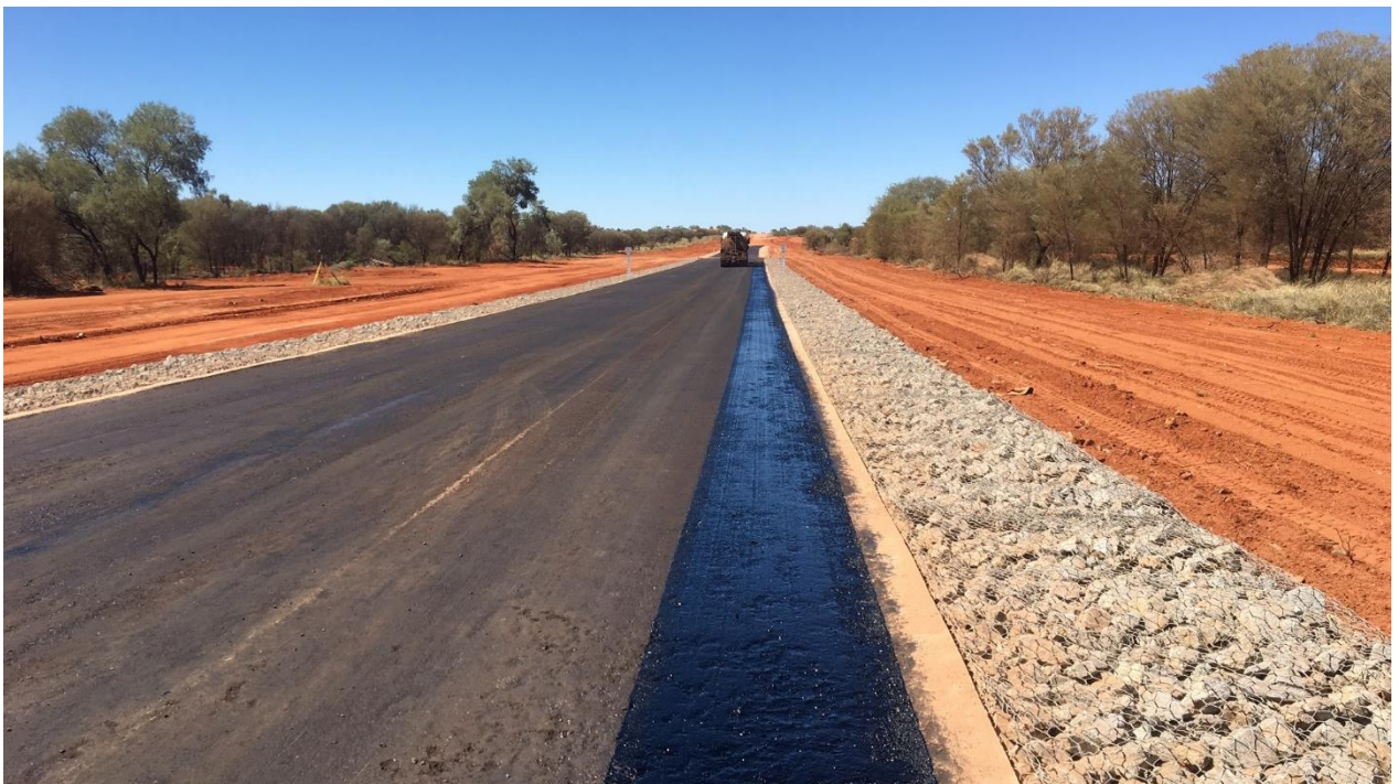
Construction photo: Maryvale Road - construct floodway at chainage 18.5 - 19.6 kilometres
