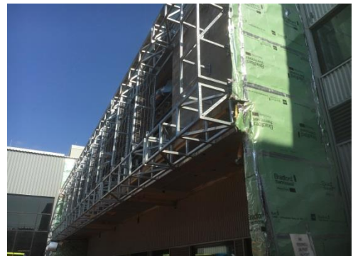
Installation of sunshade awnings to building four
