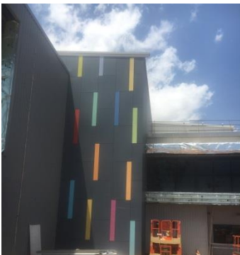
External painting works to building one
