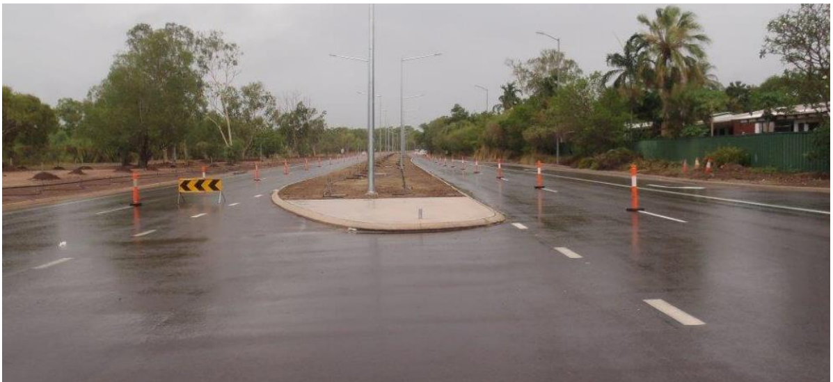
Photos: Construction works
