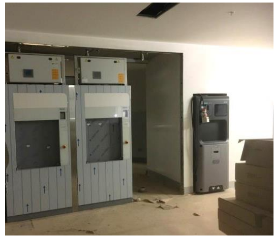
Continued installation of cabinet-washer disinfectors to CSSD
