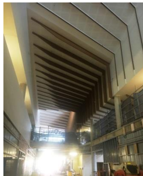
Installation of acoustic baffles to Hospital Arcade ceiling
