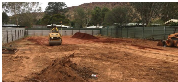
Construction photo: Gap Road
