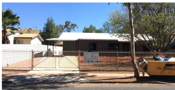
Construction photo: Lyndavale Street
