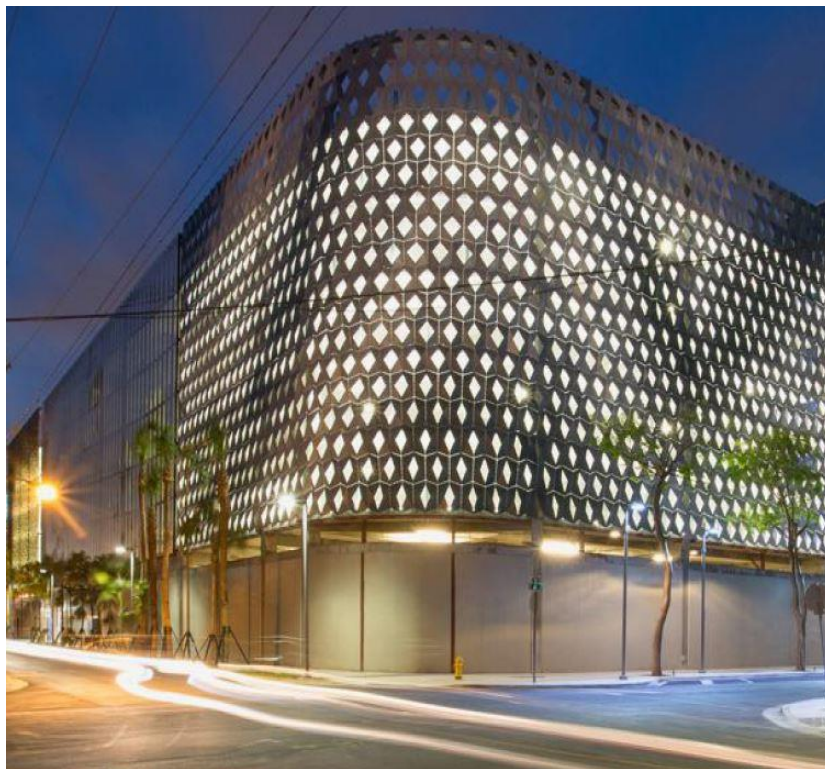
Example of façade: Palmerston CBD - 3 Mansfield Street - convert office to 98 bed student hostel plus additional roof top terrace
