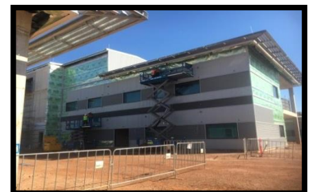
Wall cladding to south wall of building 5
