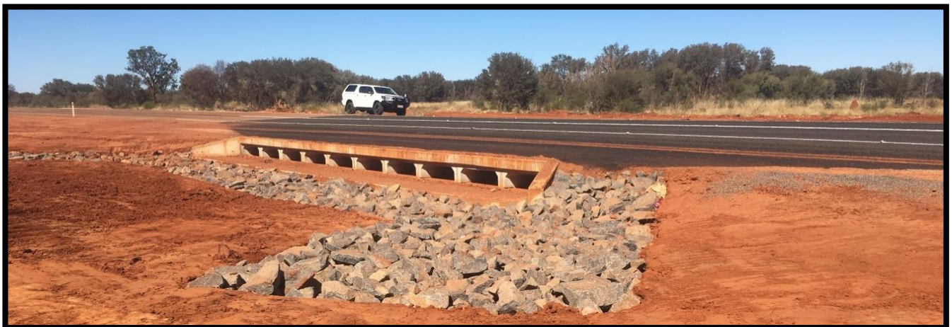
Photo: Tanami Road - upgrade and seal towards Yuendumu at chainage 252 - 257 km
