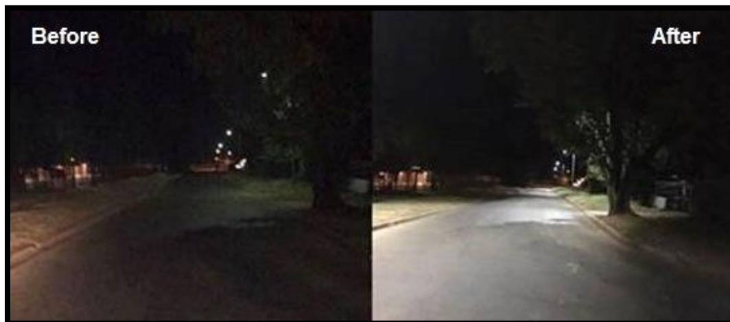
Photos: Katherine- new LED solar lighting system (example at Kirkpatrick Street)
