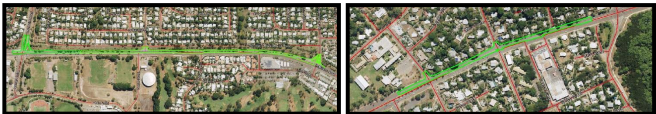
Two of various locations: Darwin Region - Northern Region - bituminous resurfacing of various roads and highways (Marrara & Millner)
