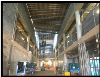
Ceiling grid to Hospital Arcade
