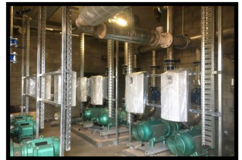
Electric motor installation to chiller plant in level 1 building 7
