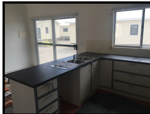
Construction Photos: Yuendumu – Government Engagement Co-ordinators – ancillary dwelling (off site construction)
