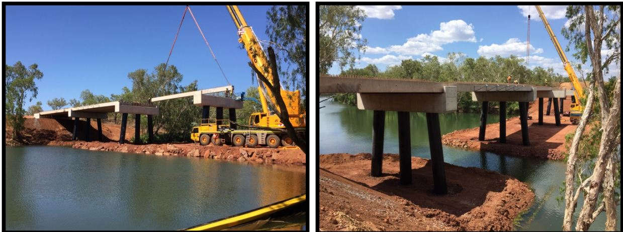
Construction Photos: Roper Highway - Roper River / Wilton River - high level bridge crossings and road upgrade
