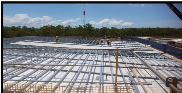
Lifting roof sheets for Building One
