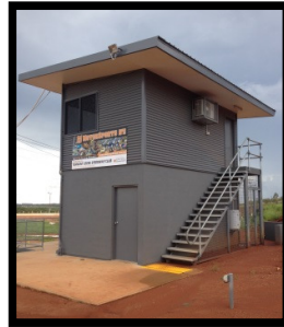
Construction Photos: Tennant Creek - Speedway
