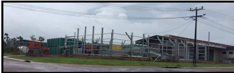
Construction Photo: East Arm - 1 Nebo Road - warehouse
