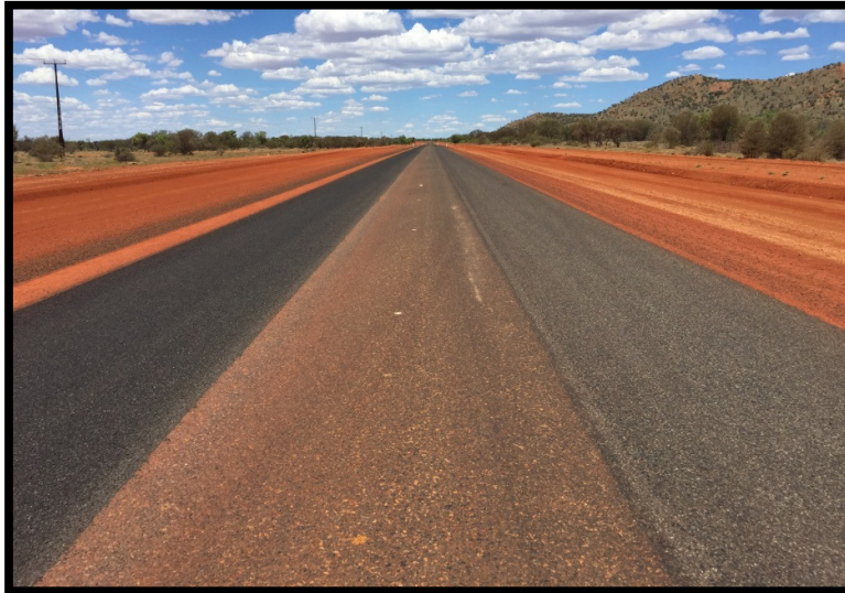
Construction Photo: Tanami Road – upgrade and seal chainage 0 - 7.24 km and 37.2 - 45.3 km
