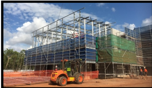
Erection of structural steel to Services Plant Room
