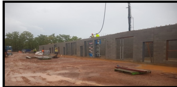
Core filling blockwork for Emergency Services Building
