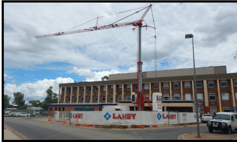
Construction Photo: Alice Springs Hospital – fire rectification works
