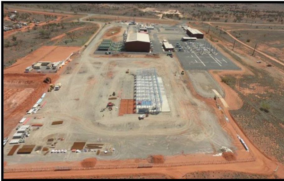
Aerial Photo: Owen Springs Power Station - power station expansion
