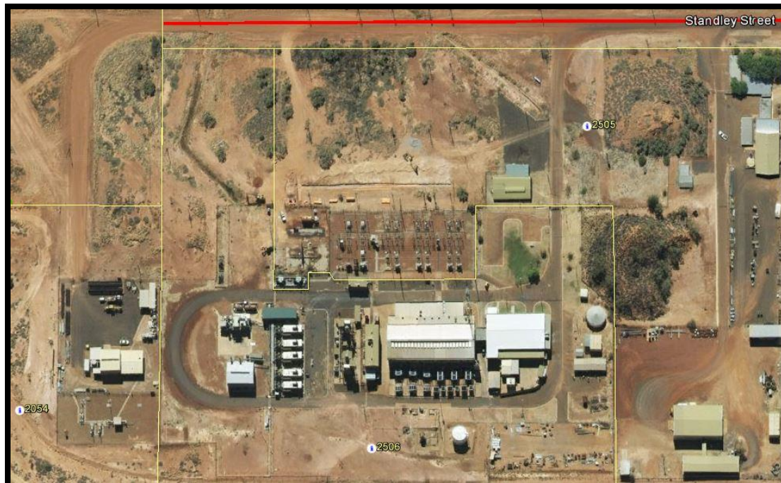
Location: Tennant Creek Power Station - power station upgrade
