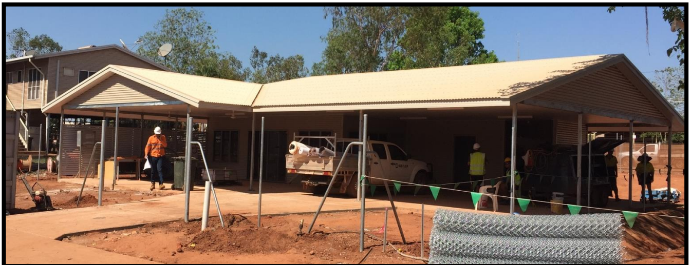
Construction Photos: Wadeye - multi purposes Police Station and accommodation
