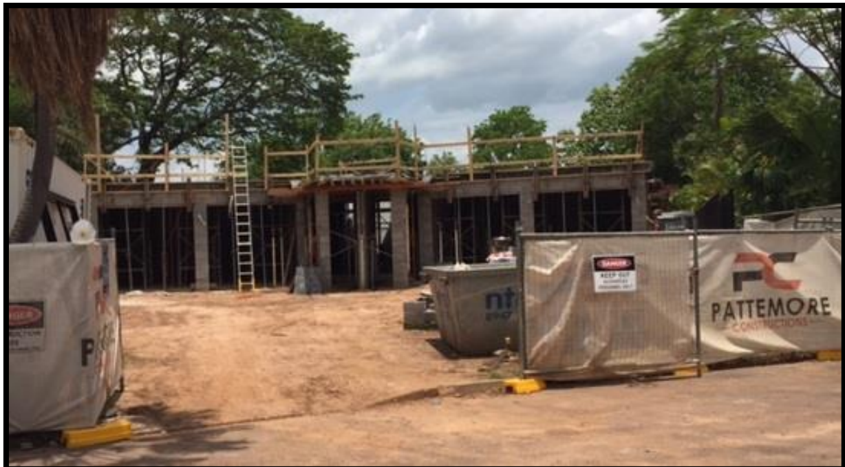
Construction Photo: The Narrows – 34 Wilmot Street – 2 by 4 bedroom townhouses
