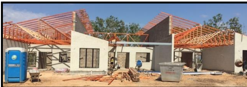
Construction Photo: Zuccoli – 4 Fern Court – 3 by 3 bedroom triplex
