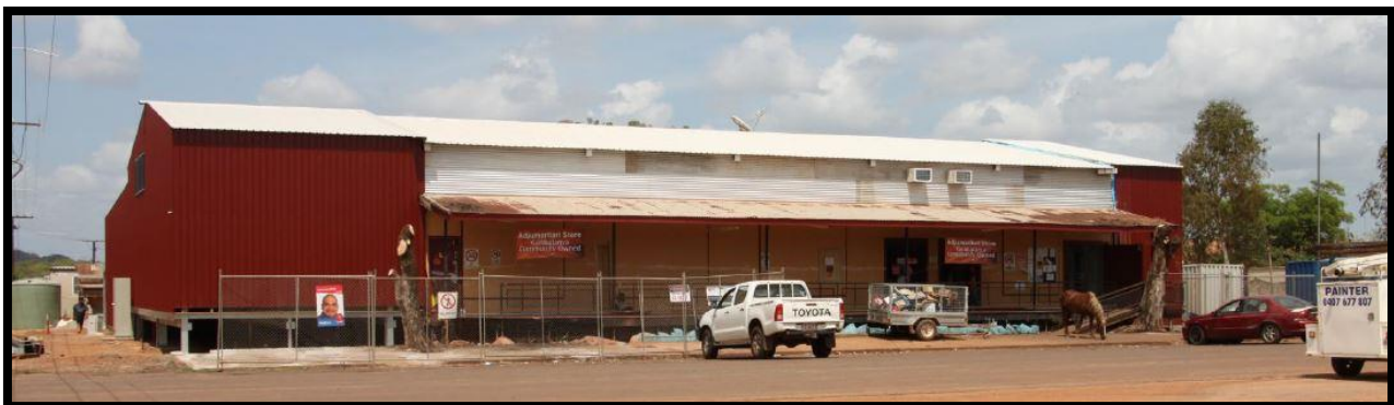
Construction Photo: Gunbalanya - lot 651 - alterations and additions to existing store
