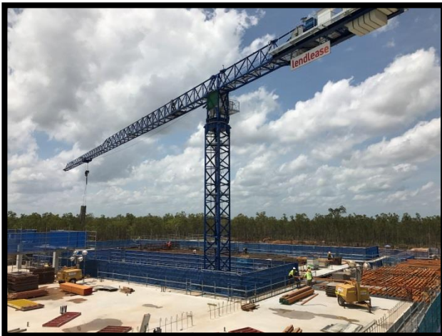
Construction Photos: Palmerston Regional Hospital (PRH)
