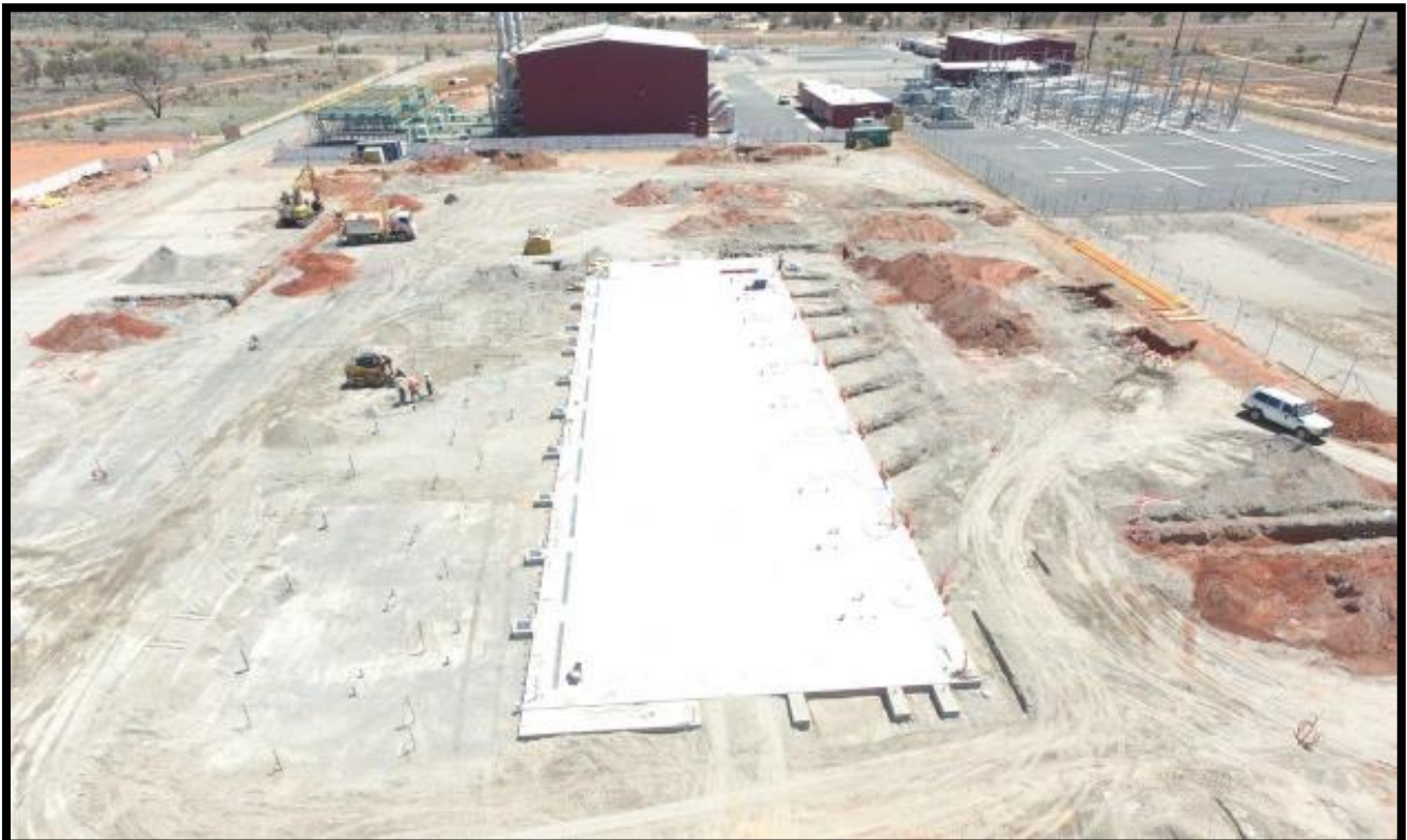
Construction Photo: Owen Springs Power Station - power station expansion
