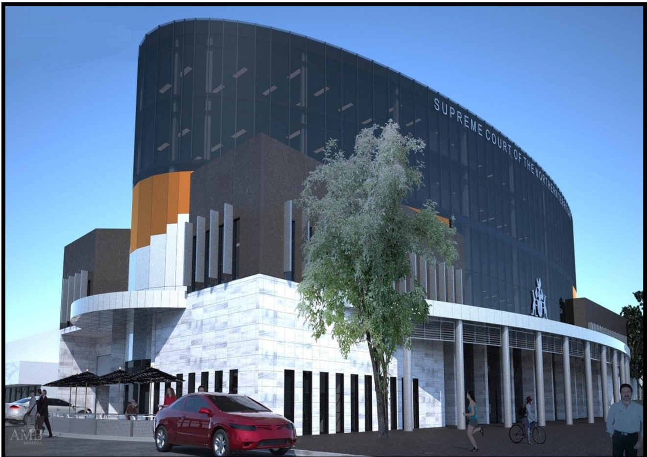
Concept Image: Alice Springs - Parsons Street - new Supreme Court and office building
