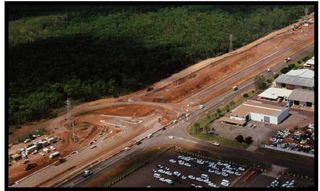
TBD at Charles Darwin / Bowen Street intersection
