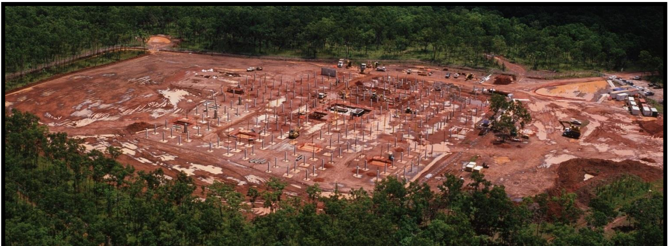
Photos: Palmerston Regional Hospital (PRH)
