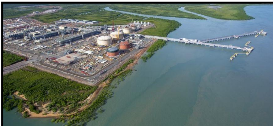
Photo: INPEX – Ichthys LNG Project onshore facilities construction continues, Bladin Point near Darwin
