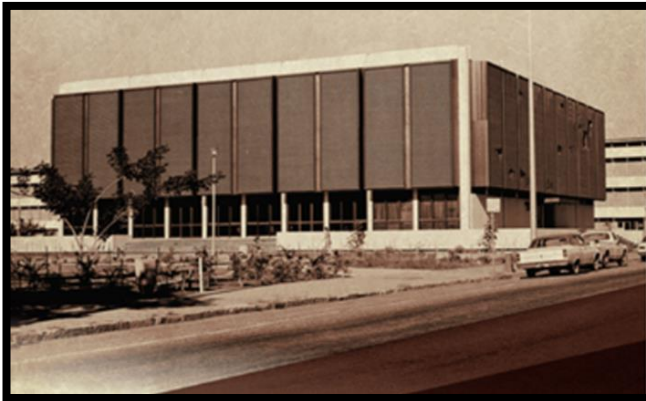
Photo: Chan Building, 1975 (damage from Cyclone Tracey still visible)
