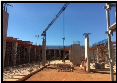
PRH – tower crane in operation
