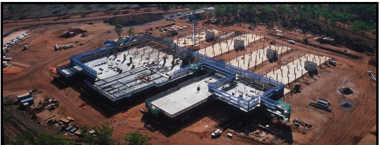
Palmerston Regional Hospital – aerial view
