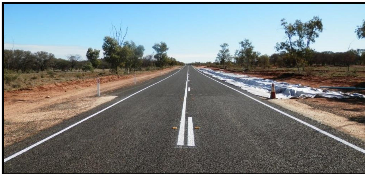
Construction Photo: Plenty Highway - chainage 140 - 146 km - upgrade and seal (stage 2)
