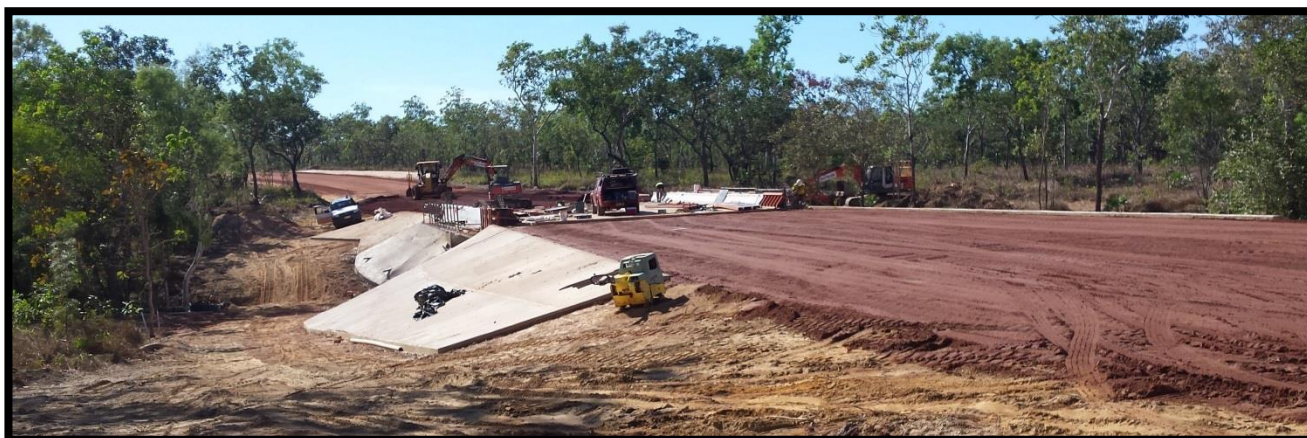
Construction Photo: Fog Bay Road - Leviathan Creek Crossing upgrade
