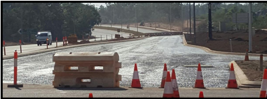
Photo: Roystonea Avenue / Temple Terrace intersection upgrade
