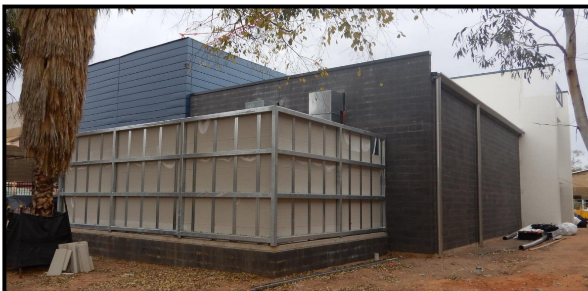
Construction Photos: Alice Springs Hospital - teaching and training facility
