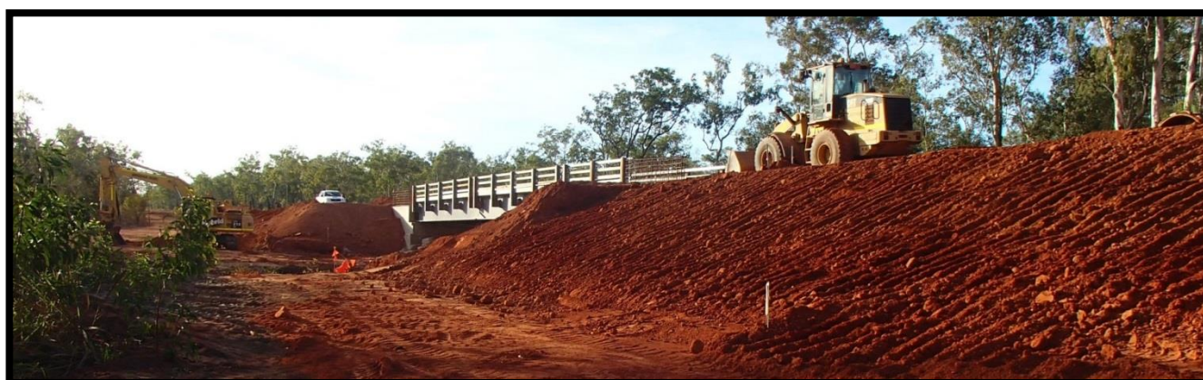
Construction Photo: Central Arnhem Road – Rocky Bottom Creek new bridge
