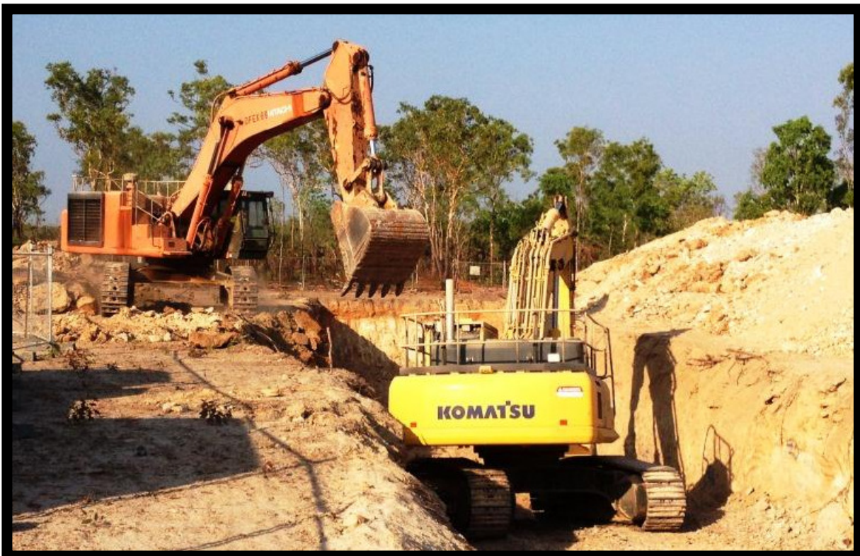
Photo: Zuccoli West Trunk Sewer project
