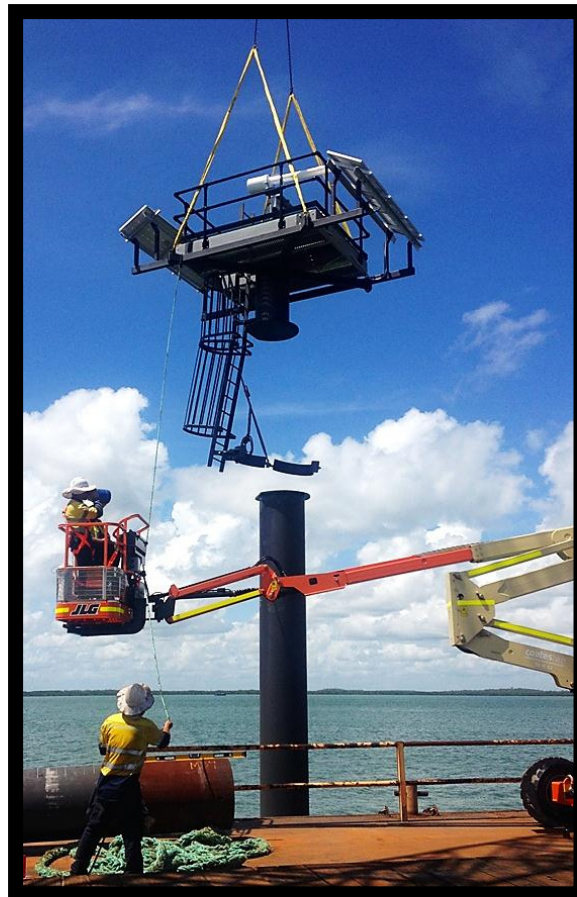
Photo: Marine Supply Base installation of navigation aid
