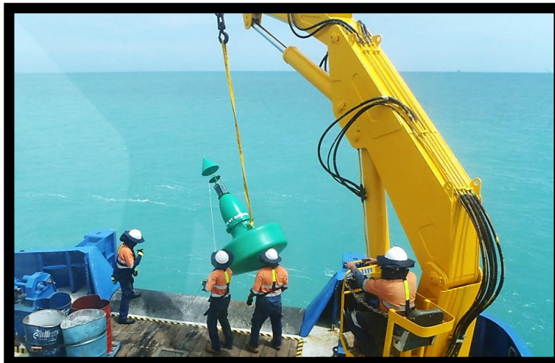
Photo: Installation of marine navigation aids in Aspley Strait
