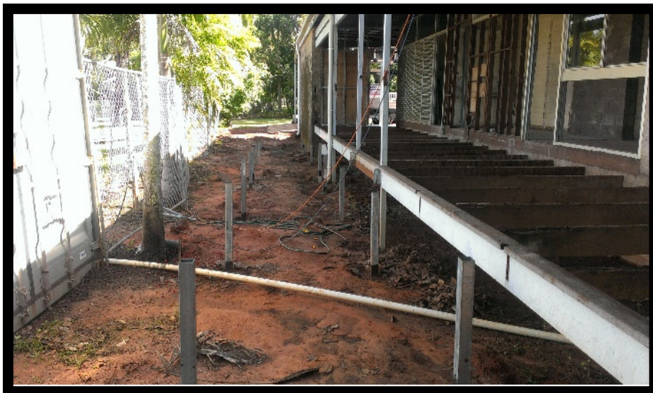
Photo: New ramp footings installed at Pirlangimpi Police Station
