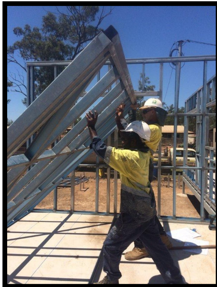
Photo: Construction of duplex, Angurugu
