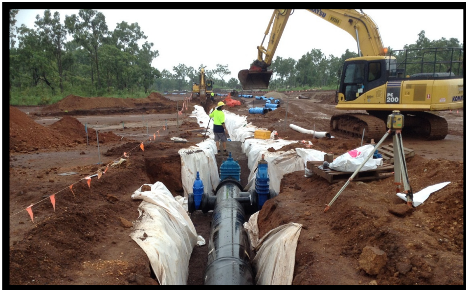
Photo: Construction of Jenkins Road water main
