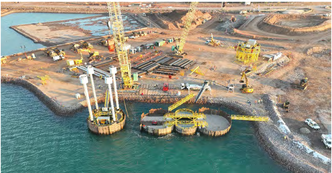
East Arm - Darwin Ship Lift Facility. Credit: Clough-BMD Joint Venture
