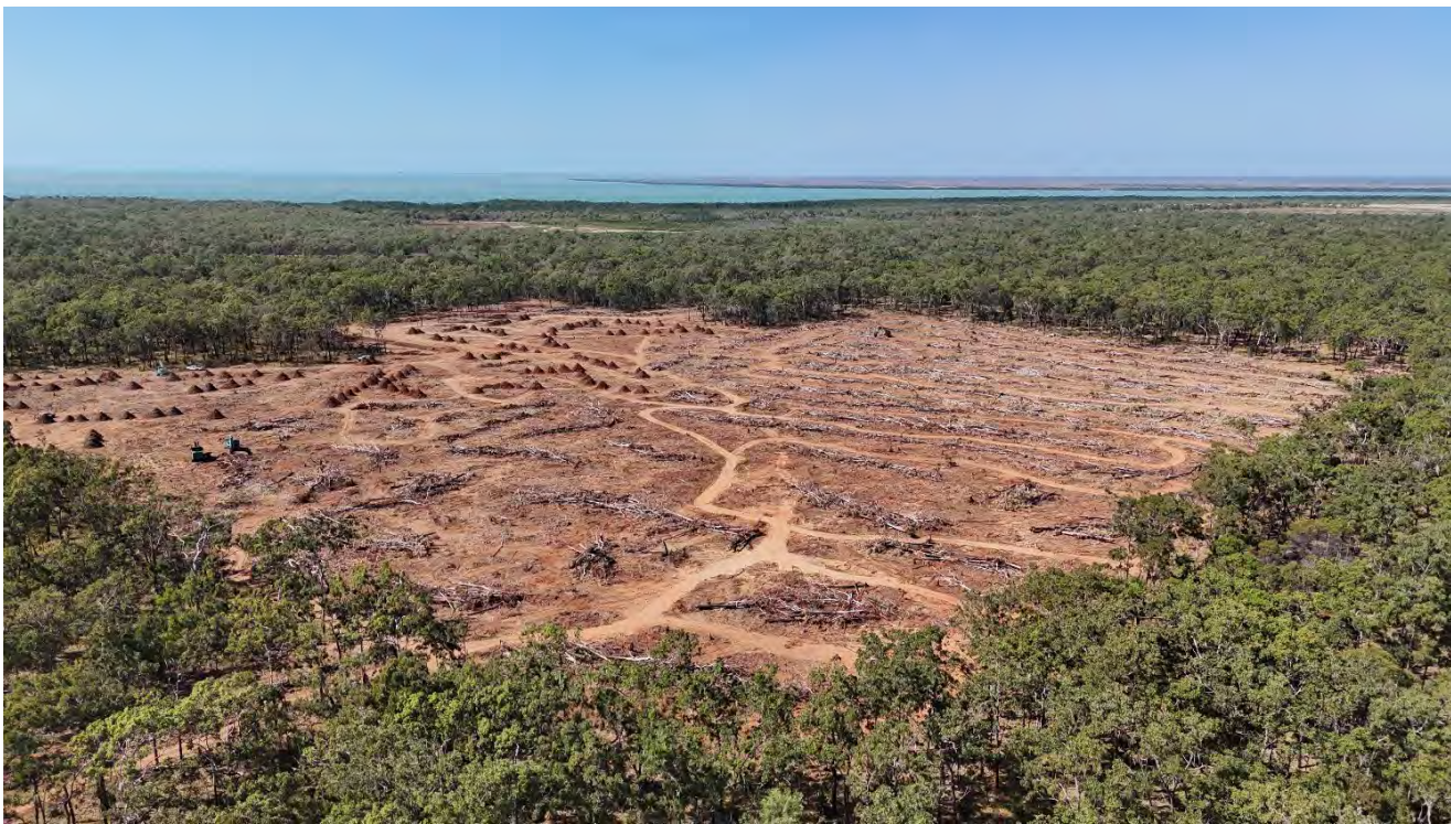
Photo: Site clearing for the Milingimbi subdivision
