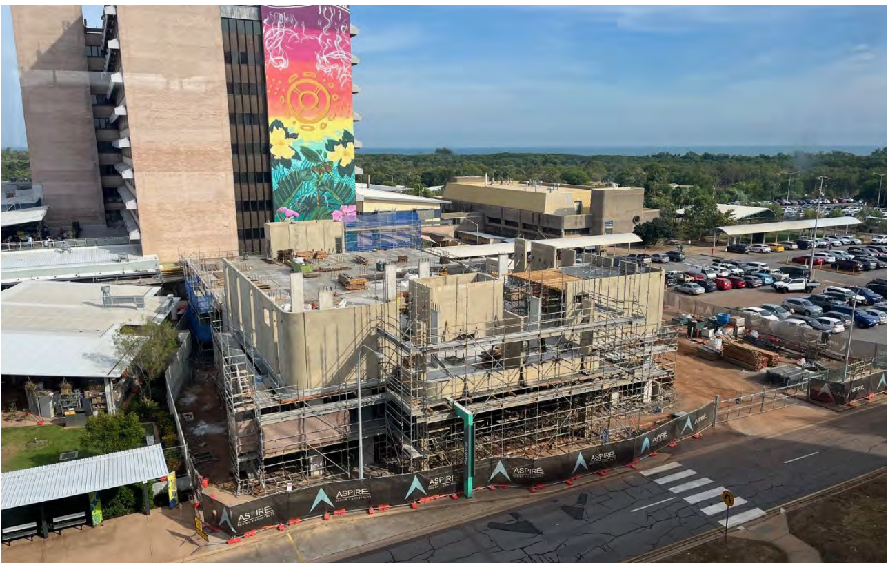
Royal Darwin Hospital - new 32 bed ward facility with 2 levels of carpark
