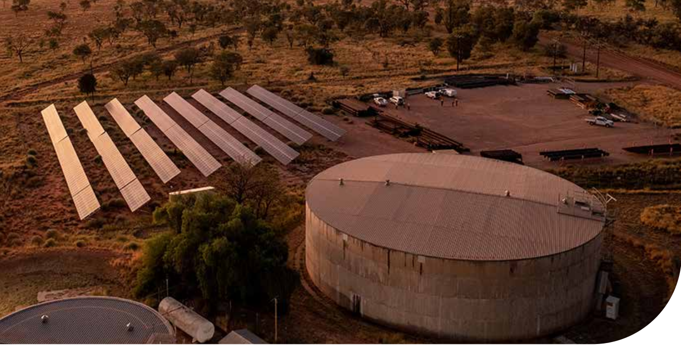
Above: Roe Creek 8 Mega Litre Water Tank. Credit: The Power and Water Corporation.
