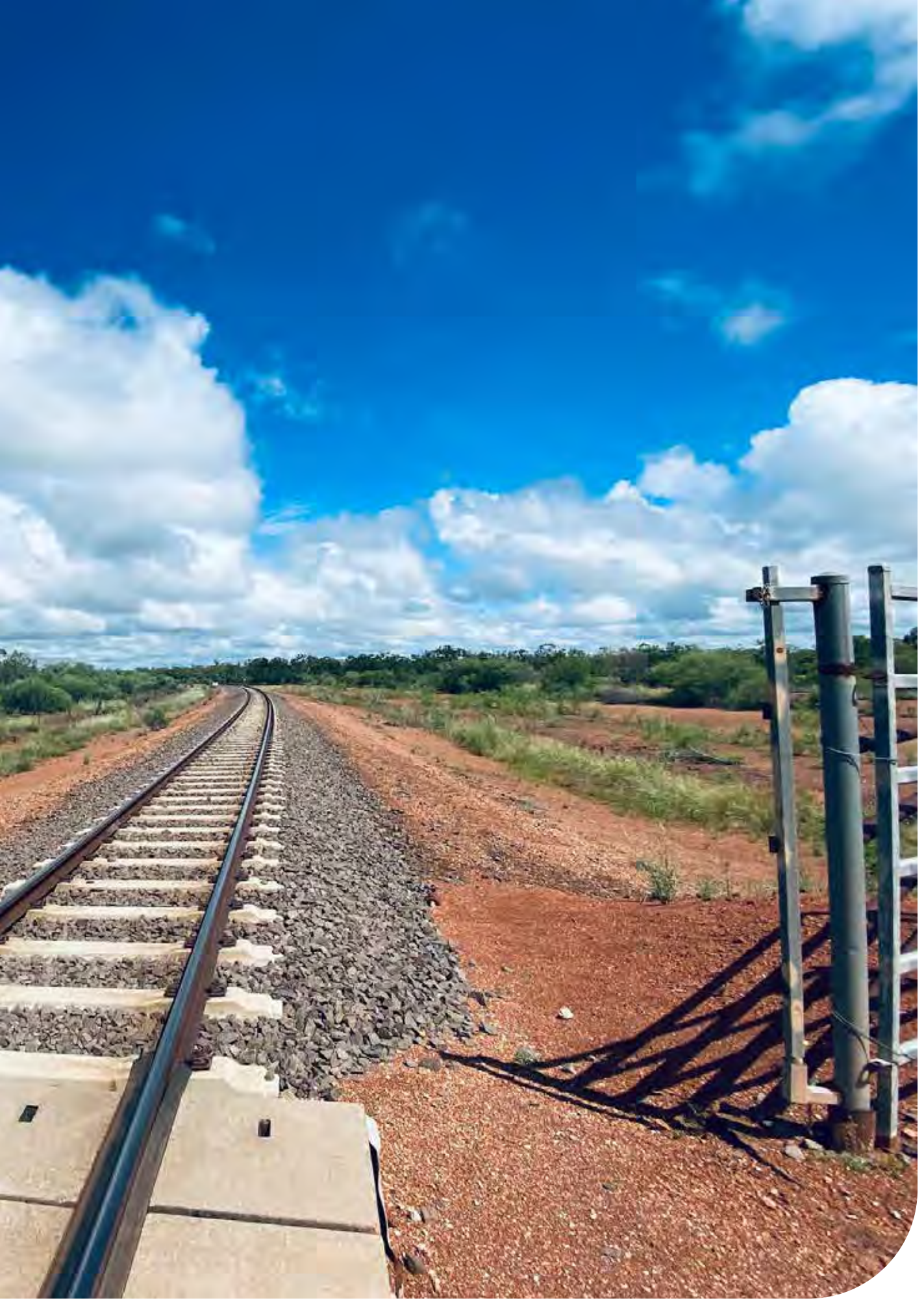
Above: NT rail line. Credit: Department of Infrastructure, Planning and Logistics.
