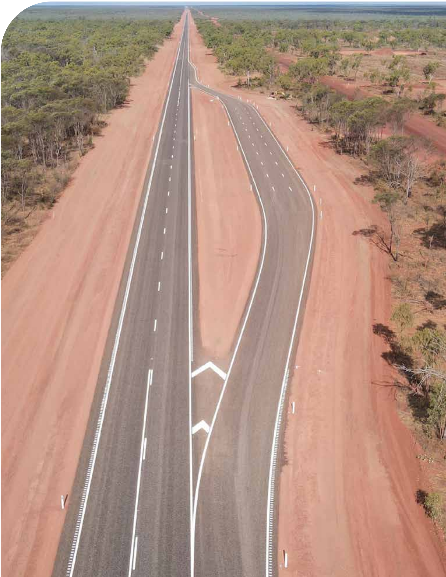
Above: Carpentaria Highway. Credit: Exact Contracting.
