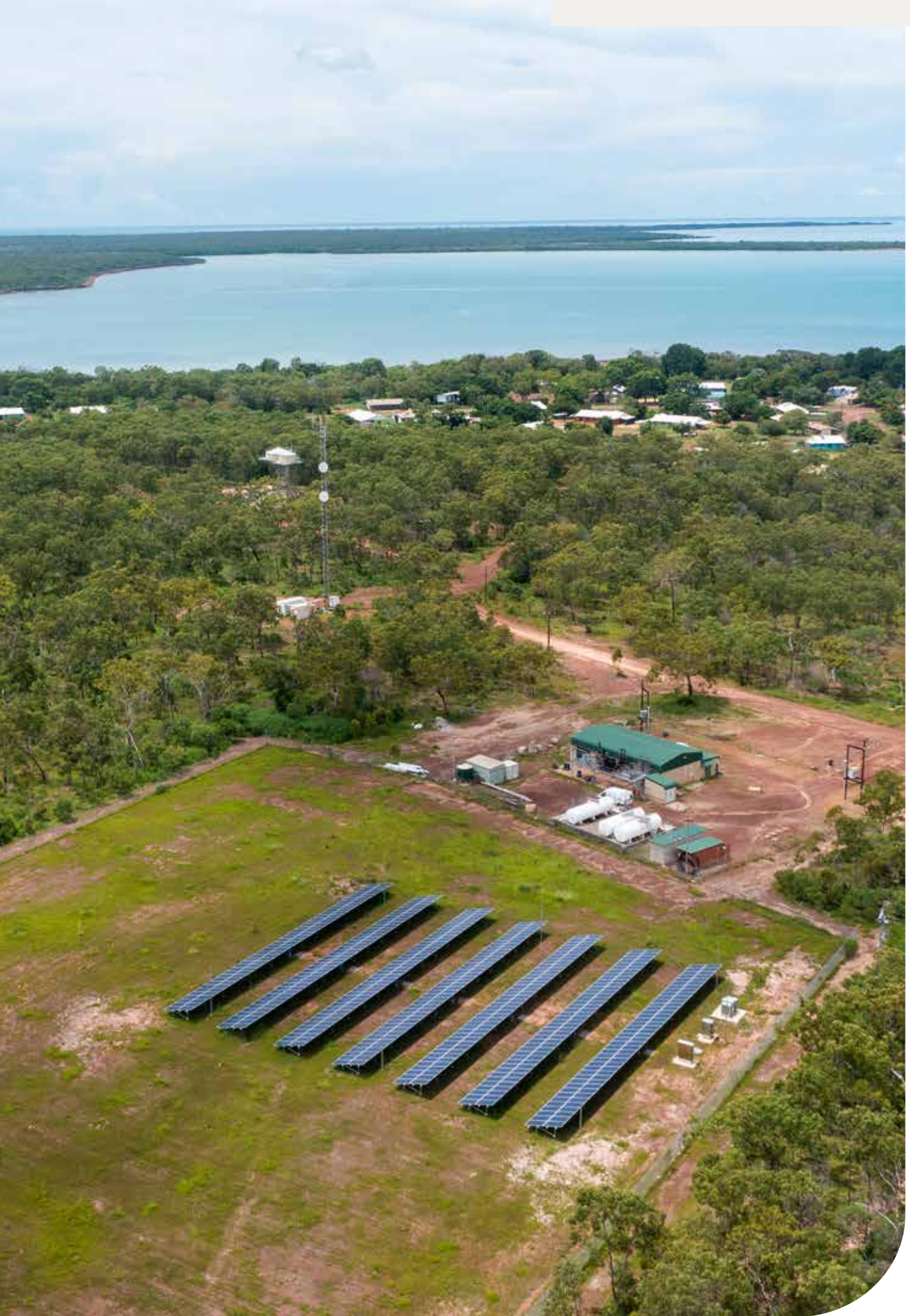
Above: Warruwi solar array. Credit: Power and Water Corporation.
