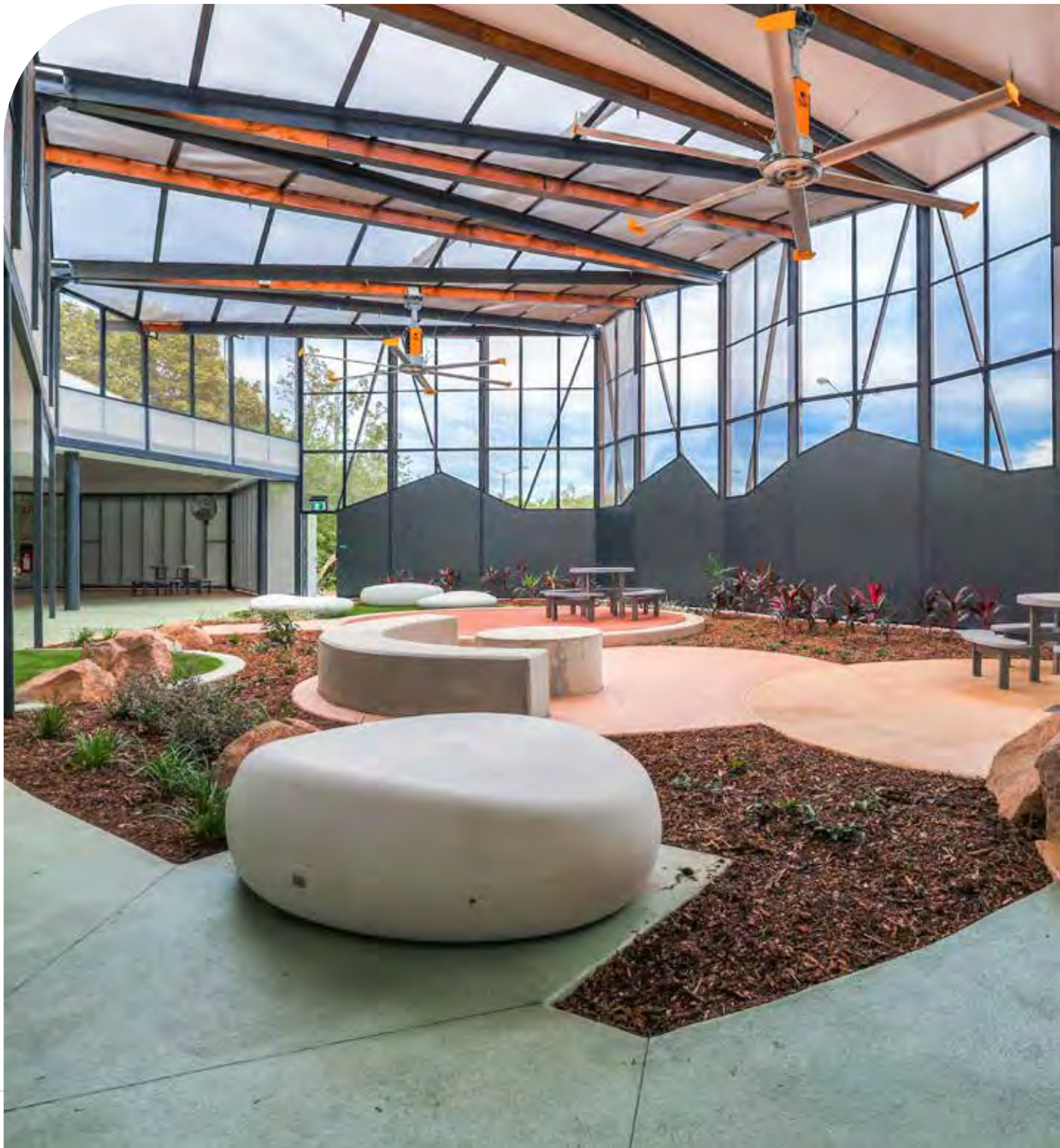
Below: Royal Darwin Hospital – Mental Health Inpatient courtyard upgrades. Credit: C & R Constructions.
