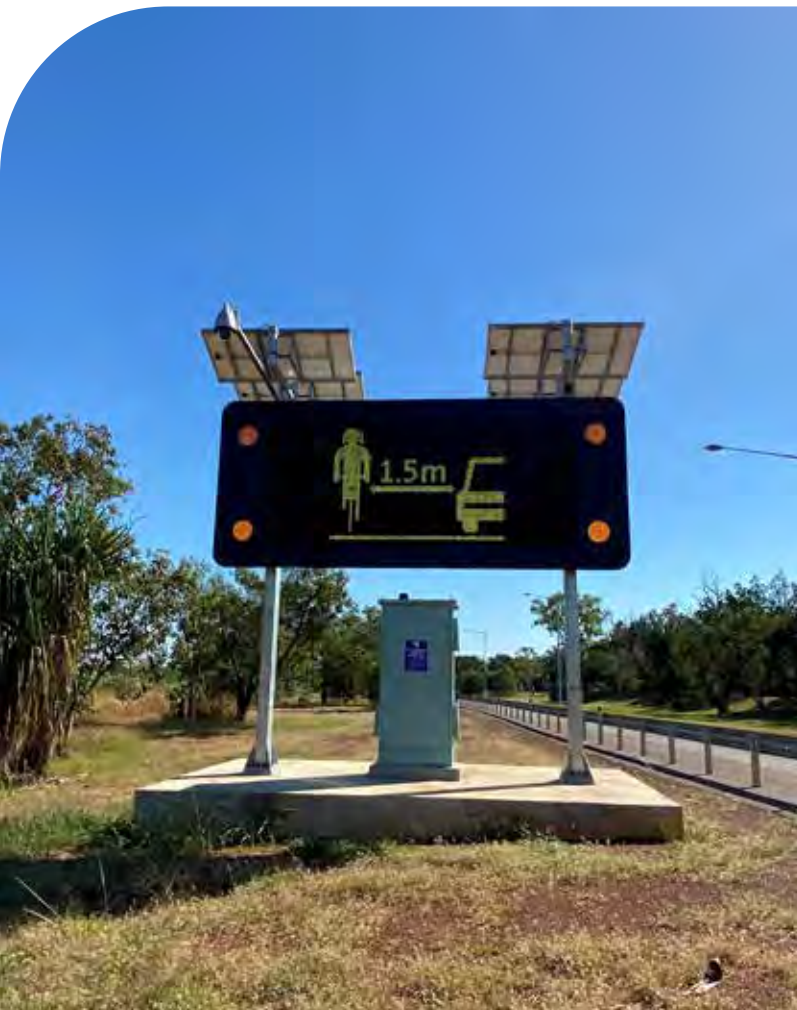
Above: Variable message board. Credit: Department of Infrastructure, Planning and Logistics
