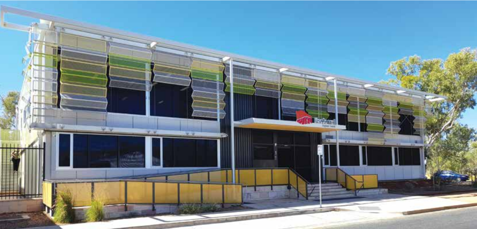
Above: MacDonnell Regional Council offices. Credit: Simon Murphy.
