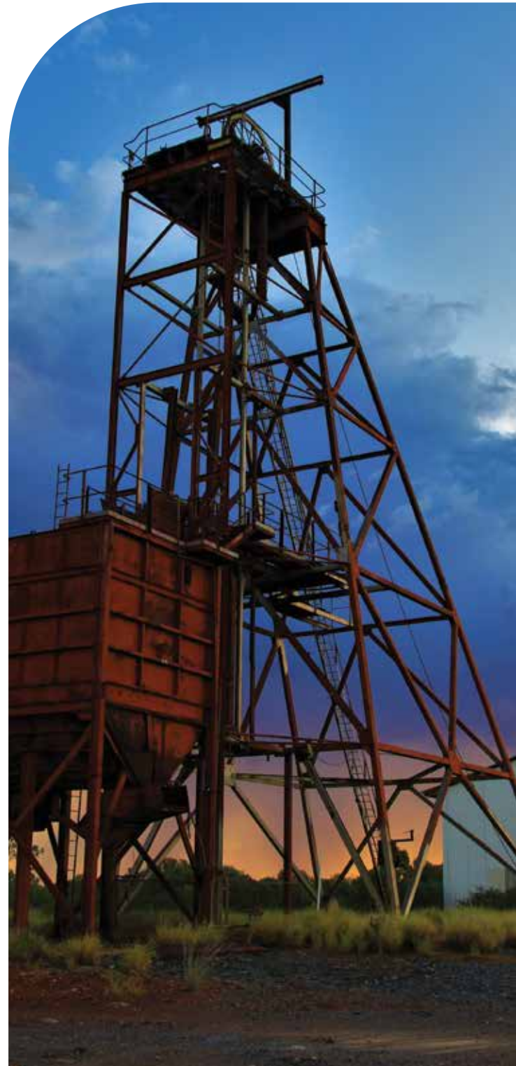
Above: Gold mining infrastructure Tennant Creek. Credit: Efsta Konidaris.
