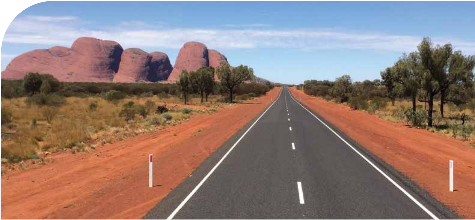
Above: Tjukururu Road. Credit: Department of Infrastructure, Planning and Logistics.
