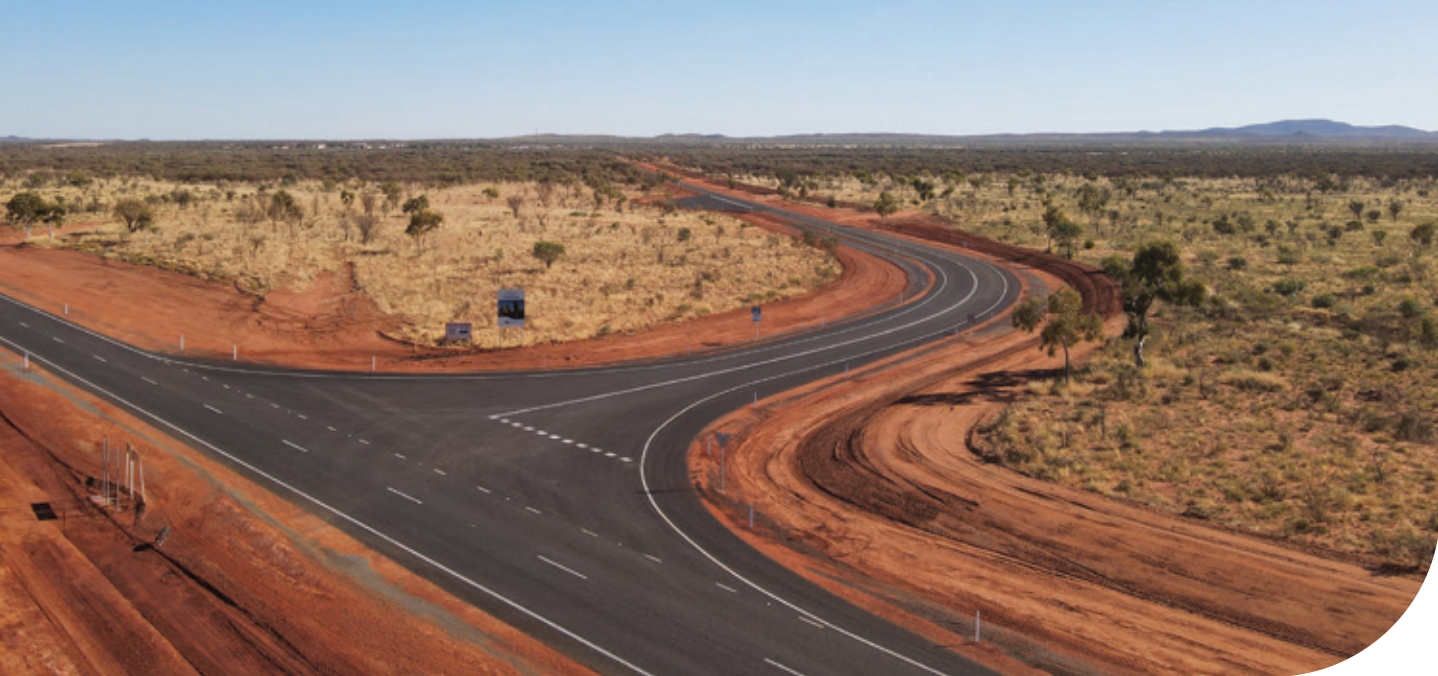
Above: Tanami Road, completion of the seal to Yuendumu turn off. Credit: Department of Infrastructure, Planning and Logistics.
