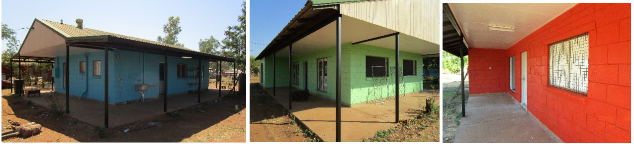
Construction photos: Robinson River - construct 4 new dwellings and upgrade 21 dwellings
