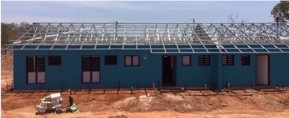
Construction photos: Rittarangu - replace 4 dwellings
