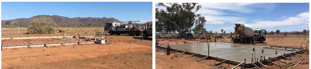
Construction photos: Atitjere - design, document and construct 3 bedroom duplex
