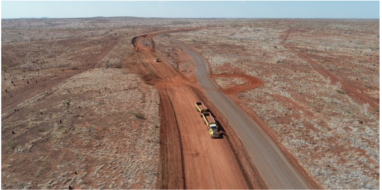
Construction photo: Buntine Highway - pavement strengthening and widening from chainage 237 - 243 km
