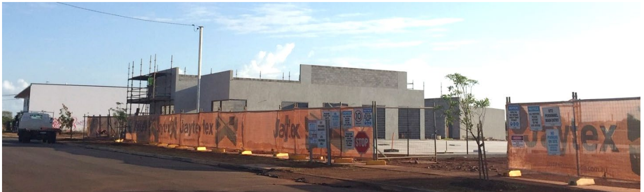
Construction photo: 18 Vaughn Street - warehouse, ancillary office and caretaker
