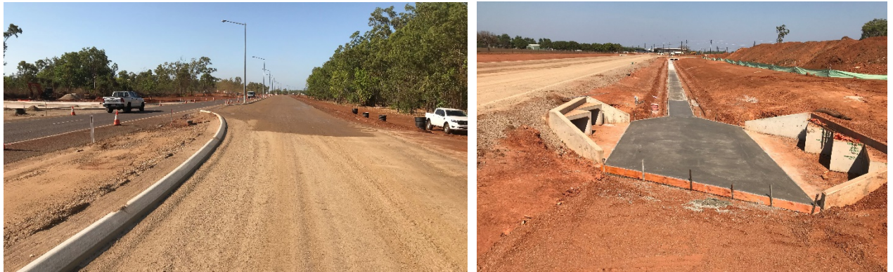
Construction photos: Berrimah - Flightpath Road - construct new road
