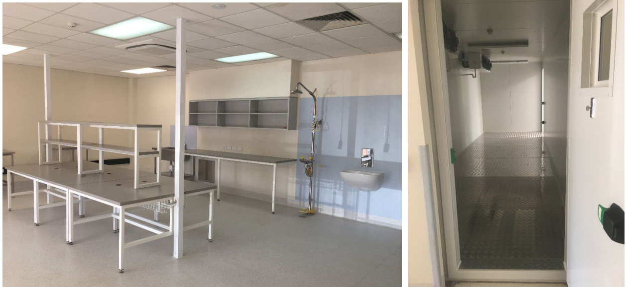
Construction photos: Alice Springs Hospital - Liebig Building pathology fit out
