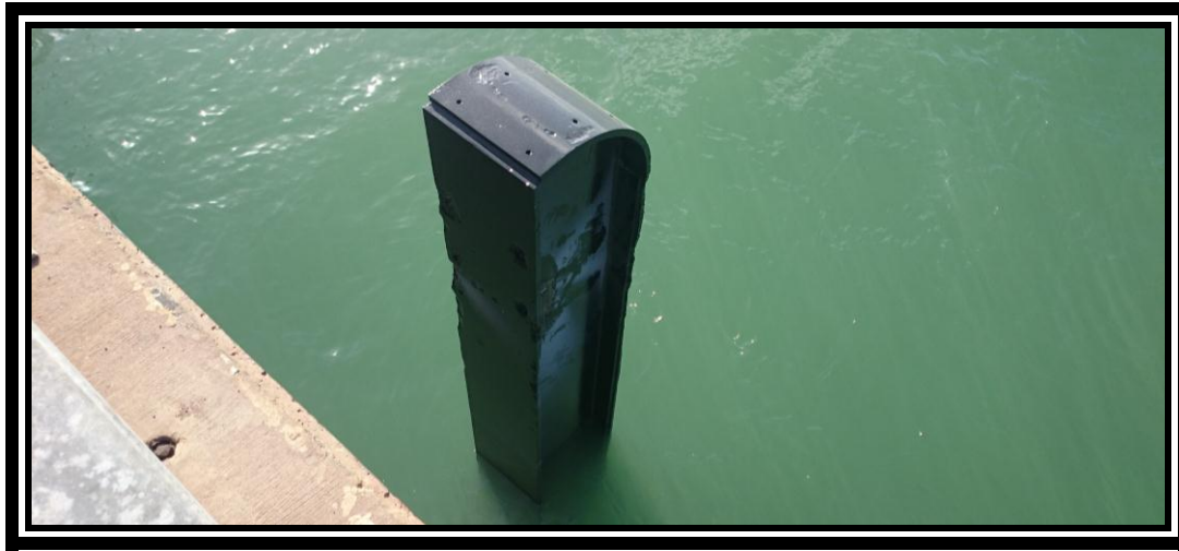
Photo: Fort Hill Wharf fender pile and whaler beam repairs
