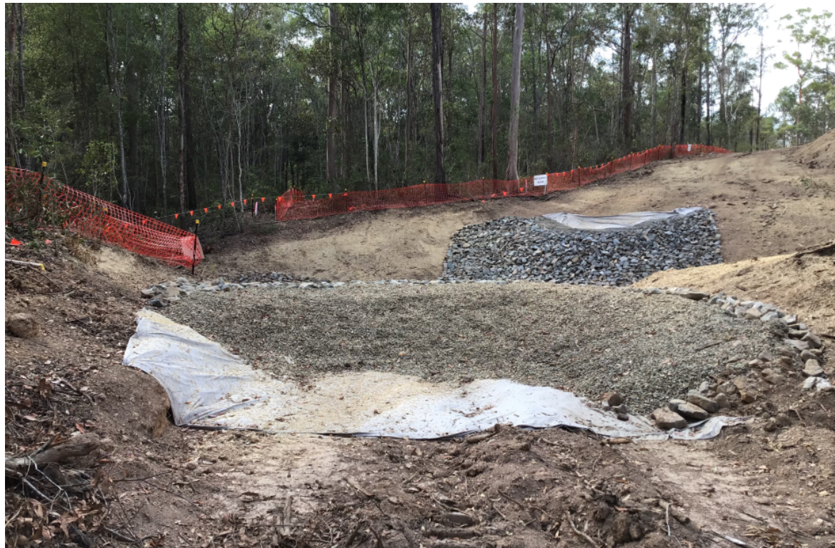
ROCK FILTER DAM (LONG SECTION)
