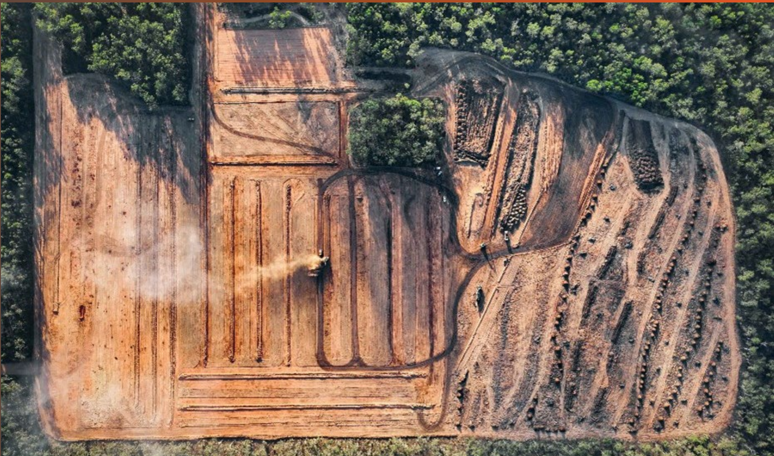
Milingimbi - Stage 1 - subdivision civil works and services construction
