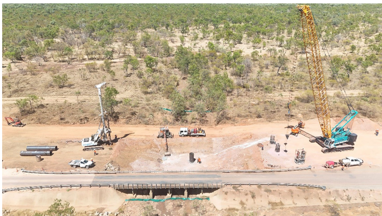
Carpentaria Highway - design and construct upgrade to 2 lane seal - 140 - 175 km including demolish and construct October Creek Bridge. Photo credit: Exact Construction
