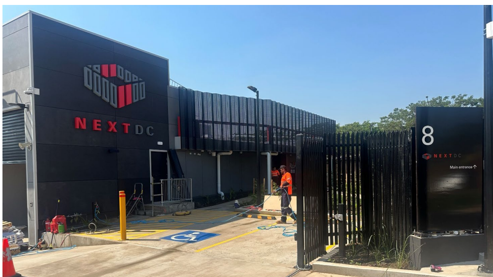
Darwin - 8 Ryko Court - NEXTDC D1 data centre. Photo courtesy of NEXTDC
