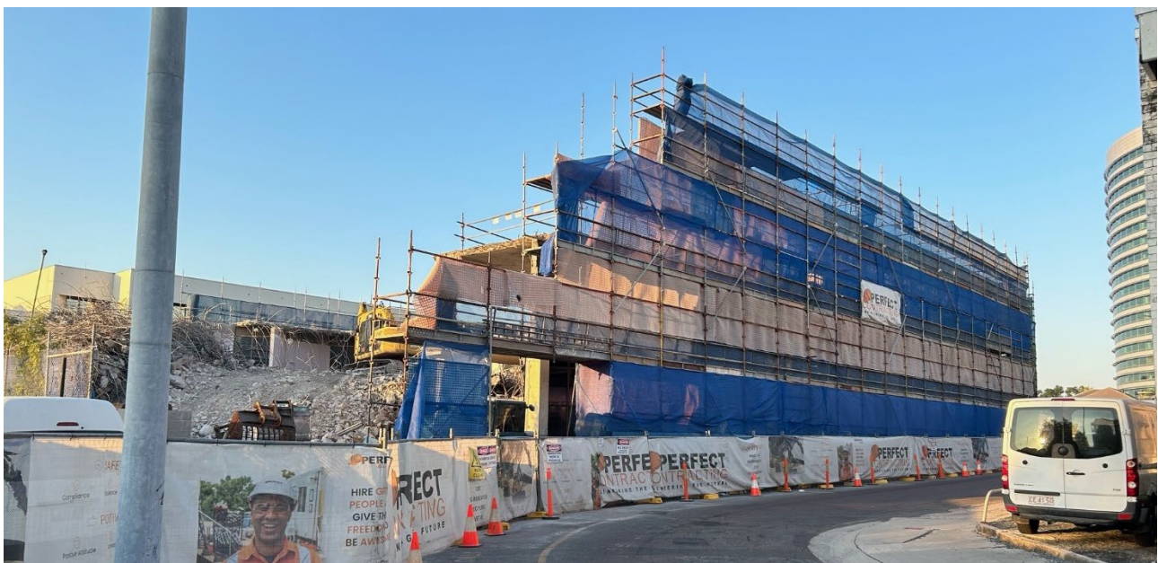
Darwin CBD - 8 Cavenagh Street – demolition
