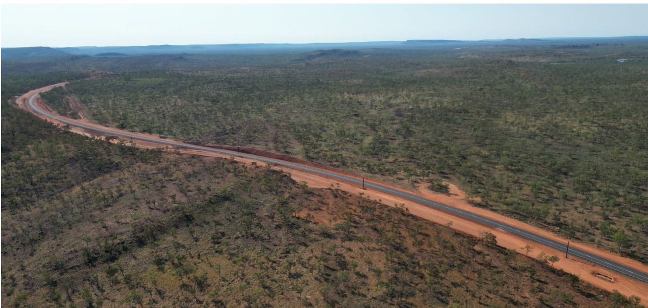
Roper Highway – upgrade to seal between 186 - 205 km
