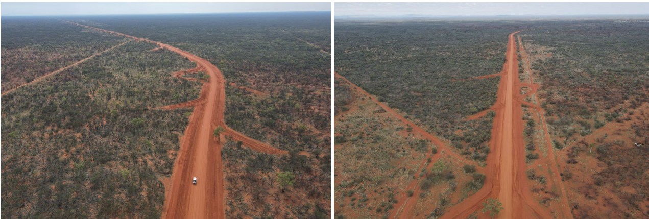
Nturiya Road – flood damage reinstatement
