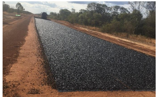
Construction photos: Carpentaria Highway - chainage 118 -121 km
