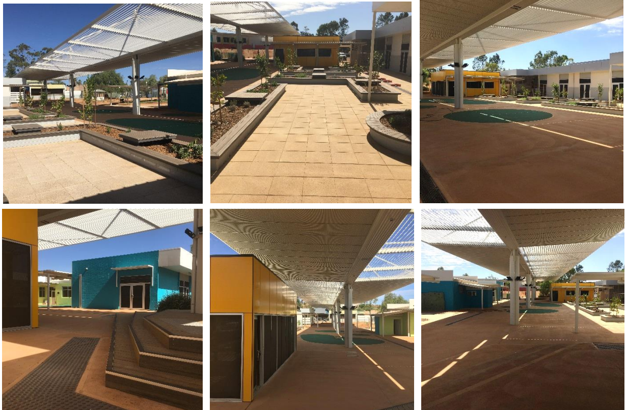
Construction photos: Braitling Primary School - Stage 2 Masterplan Works for Early Learning
