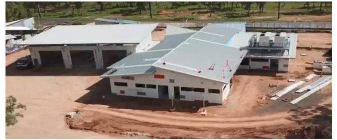
Construction photos: Katherine - Fire Station
