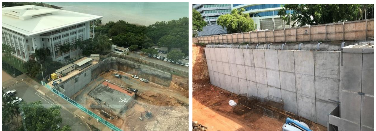
Construction photos: State Square - new 450 space underground carpark
