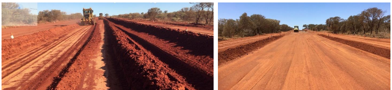
Construction photos: Tjukururu Road - upgrade and seal between chainages 8 - 12 km
