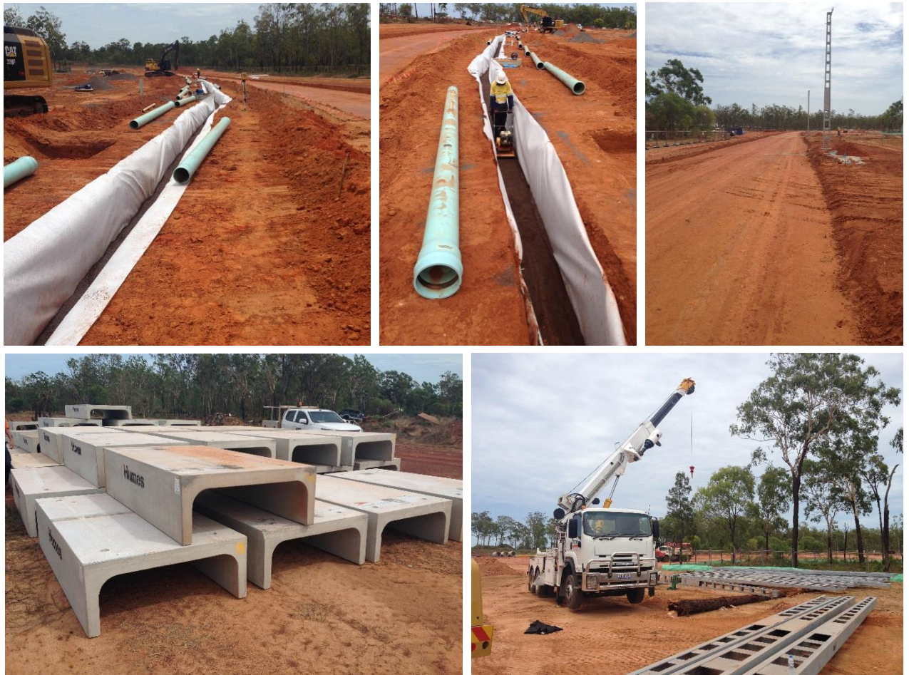
Construction photos: Maningrida - stage 1 - 30 lot subdivision civil works and services
