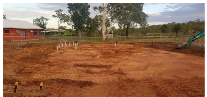
Construction photos: Minyerri - replace 14 dwellings
