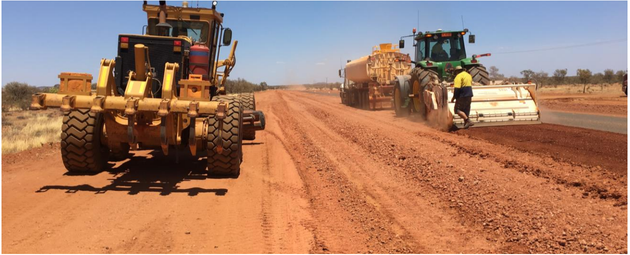
Construction photo: Tanami Road - upgrade and seal between chainage 257 - 261 km
