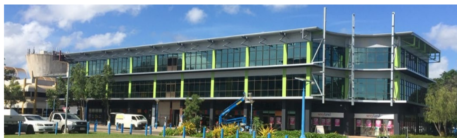
Palmerston - 3 Mansfield St - building refurbishment, restaurant fit out, office bathroom renovation and new facia
