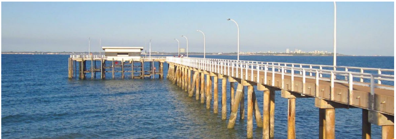
Existing infrastructure: Mandorah Marine Facilities (jetty)
