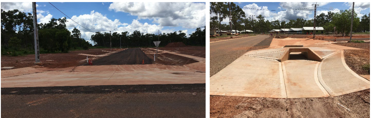
Construction photos: Lake Evella Subdivision - stages 2 & 3 - 20 lots - civil works and services
