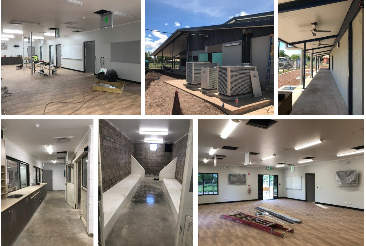
Construction photos: Angurugu - new permanent police post including multi-function area
