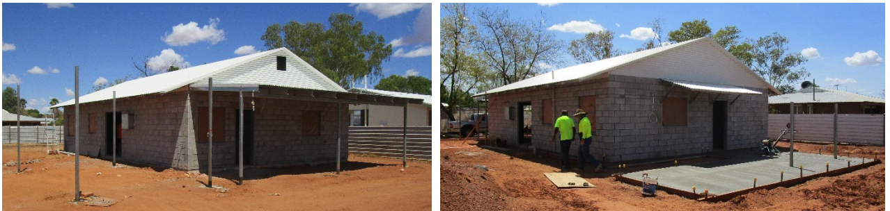
Construction photos: Tennant Creek - design, document and construct 4 by 3 bedroom dwellings
