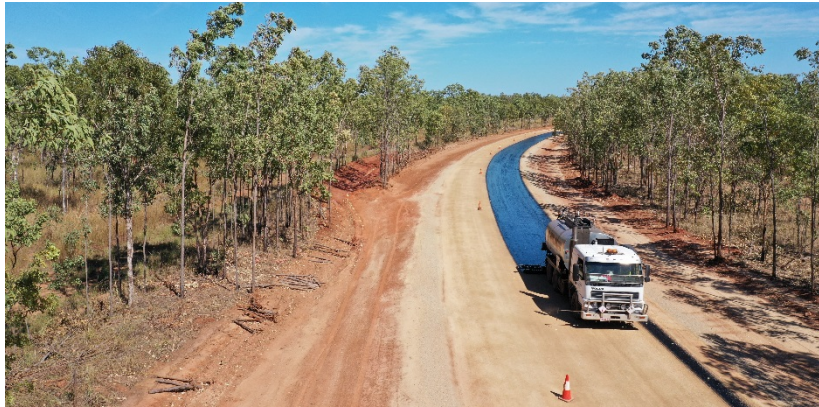
Construction photo: Beasley Road - pavement upgrade between chainage 0 - 2 km
