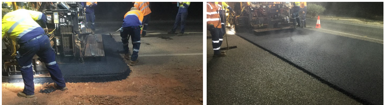
Construction photos: Yulara - upgrade 3 intersections to asphalt wearing surface
