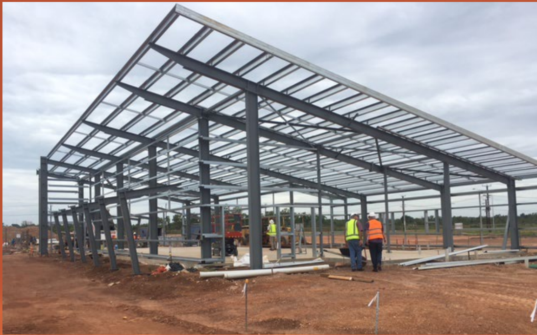
Wishart - Truck Central - heavy vehicle inspection facility
