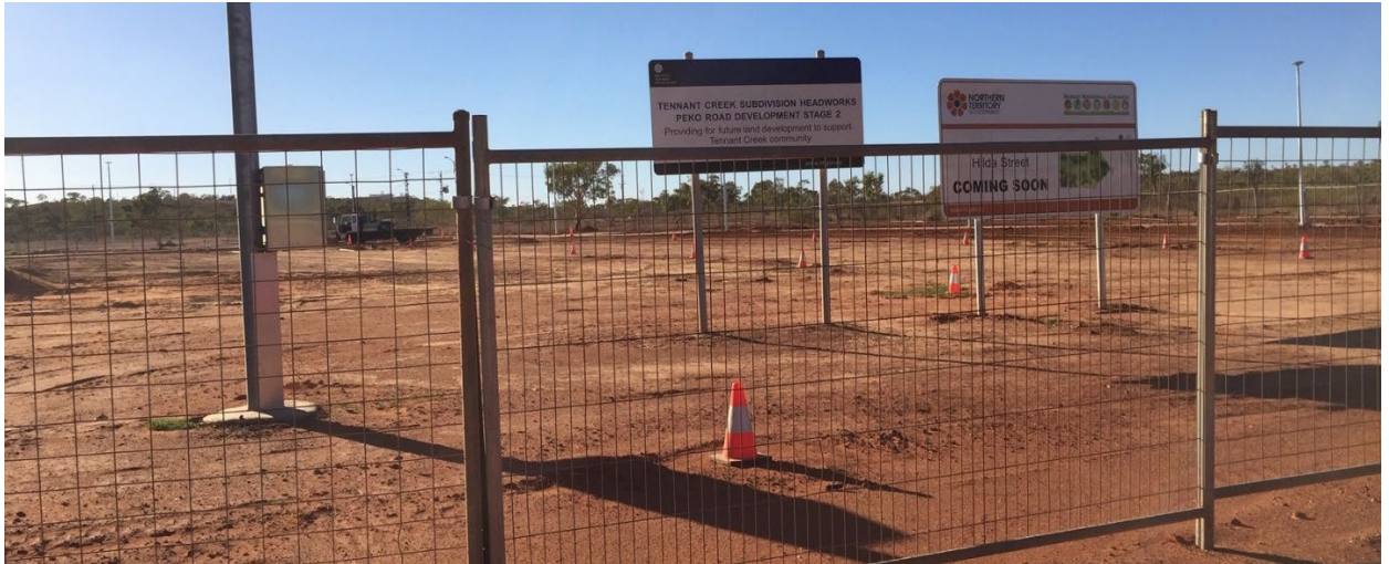
Site photo: Tennant Creek - Hilda Street - construct and landscape subdivision park
