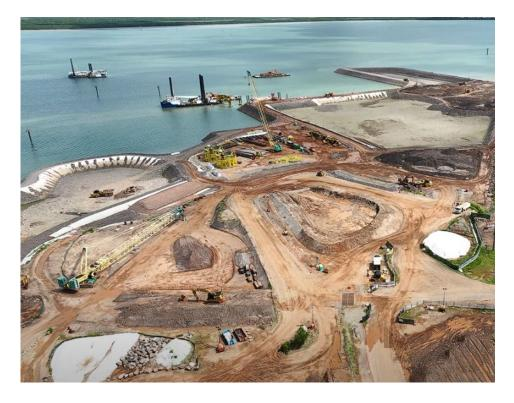
**Above:** Progress continues on the land reclamation for the Darwin Ship Lift Facility project with the caisson templates being assembled on site to start building the caissons to form the sea walls.
