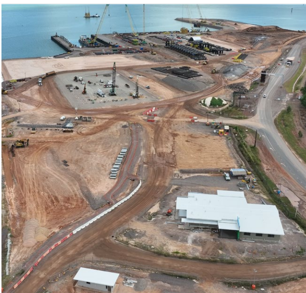
Northern Marine Complex construction site progress
