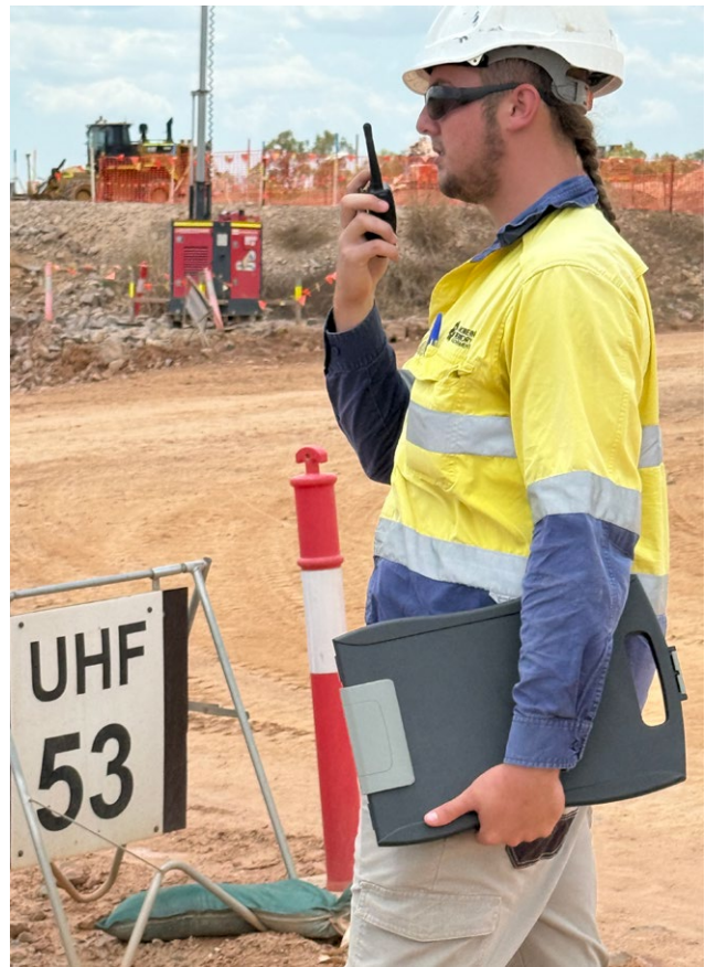
Inspections at the construction site
