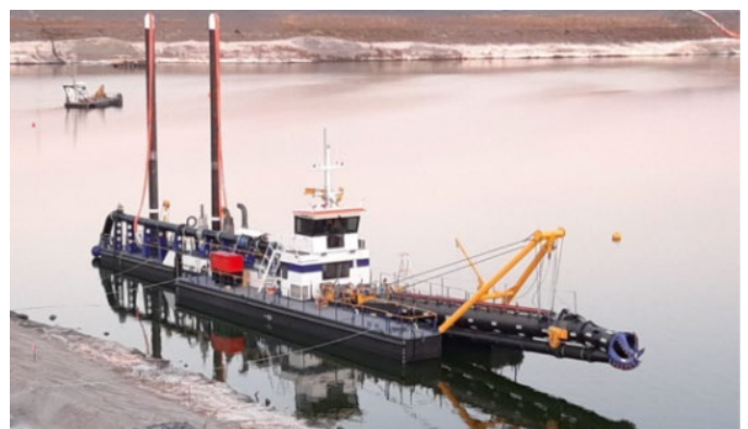
Below: Cutter suction dredger Arnhem will start dredging in late August.
