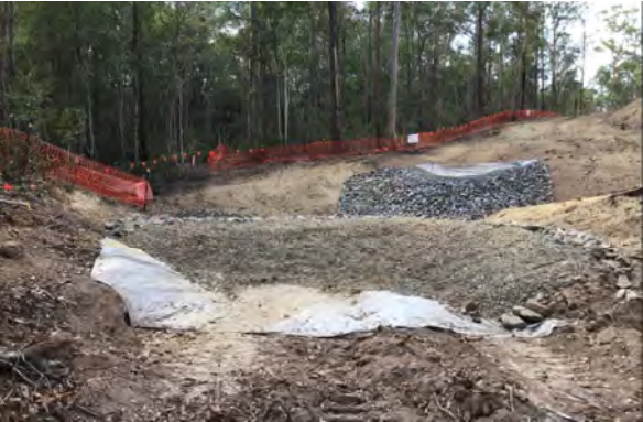
ROCK FILTER DAM (LONG SECTION)
