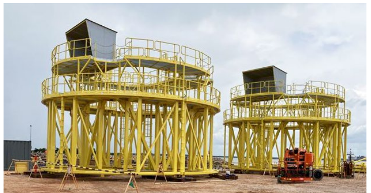
Above: Caisson templates on the ship lift facility site. Below: Example of a seawall constructed using caisson templates.
