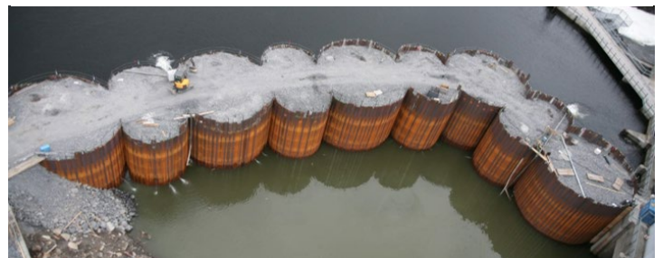
Above: Caisson templates on the ship lift facility site. Below: Example of a seawall constructed using caisson templates.
