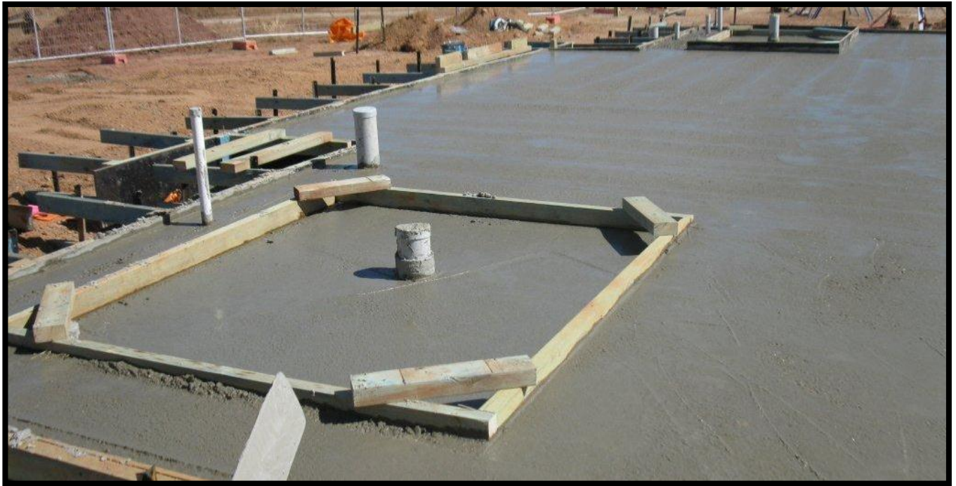
Photo: Kalkarindji - construct Government Employee Housing – concrete slab
