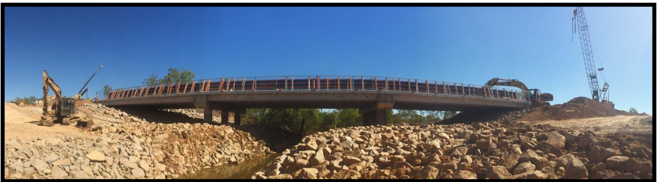
Photo: Palmerston East - Southern Connector Road and Mitchell Creek Bridge
