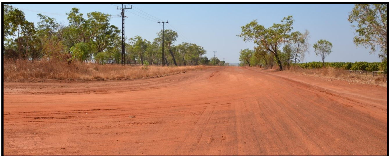
Photo: Carbeen Park Road - Katherine rural roads upgrade
