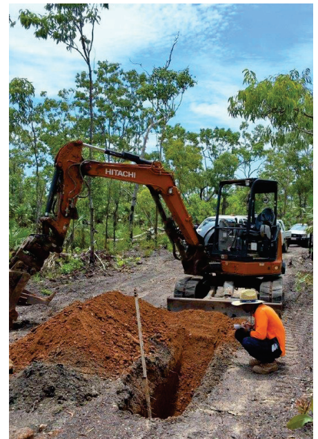
Support vehicles and site setup
