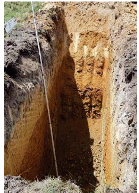
Example of excavated test pit prior to backfilling
