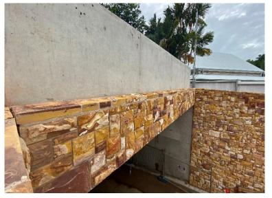
Porcellanite stone (*see image left*) has been used to line the entrance to the basement car park, with installation completed in December 2024. Local stonemason Finlay's Stone prepared and clad the basement entry using the porcellanite stone recycled from the site excavation of the gallery building.
