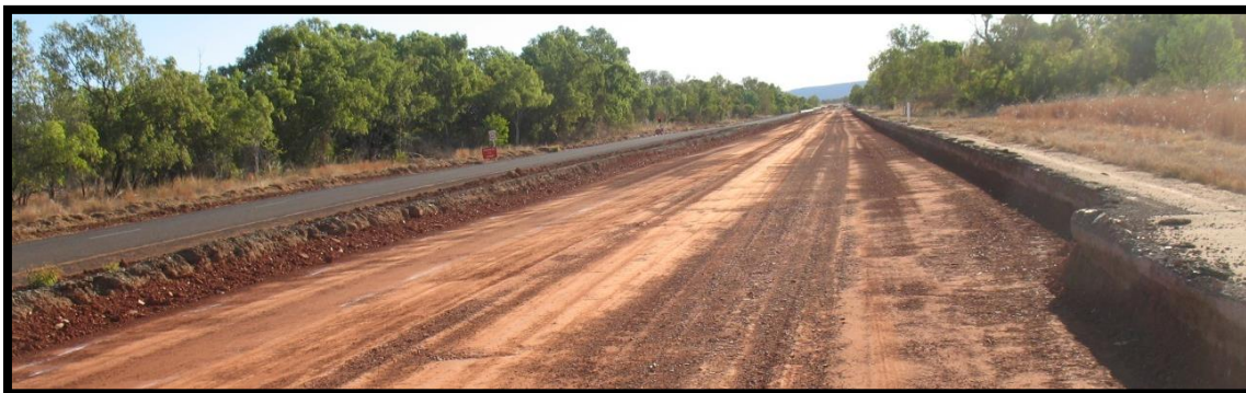
Photo: West Baines - stage 3 chainage 377 - 380km
