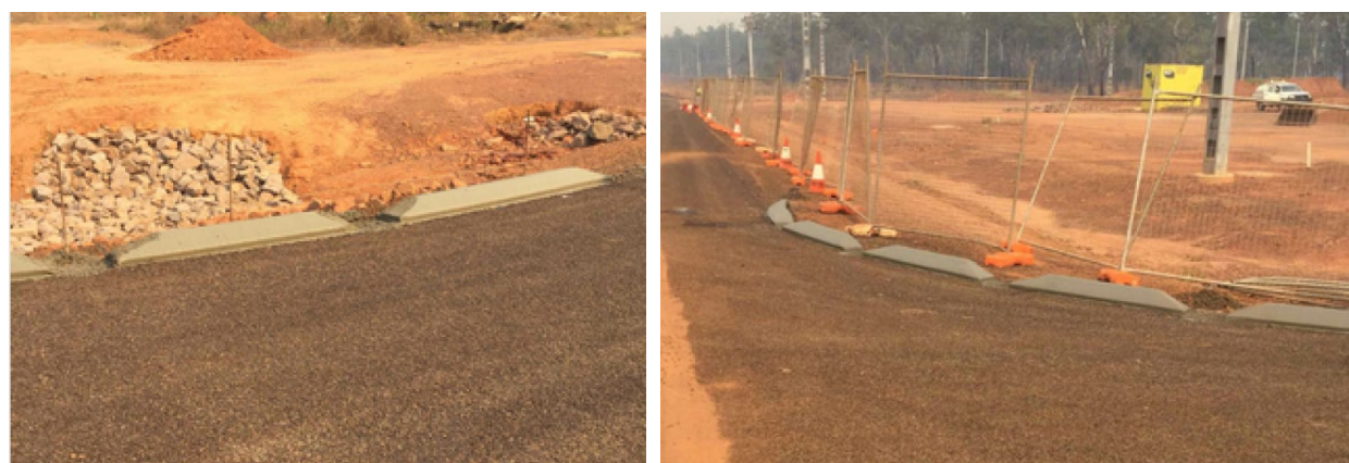
Construction photos: Wadeye - stage 1 subdivision - civil works and services
