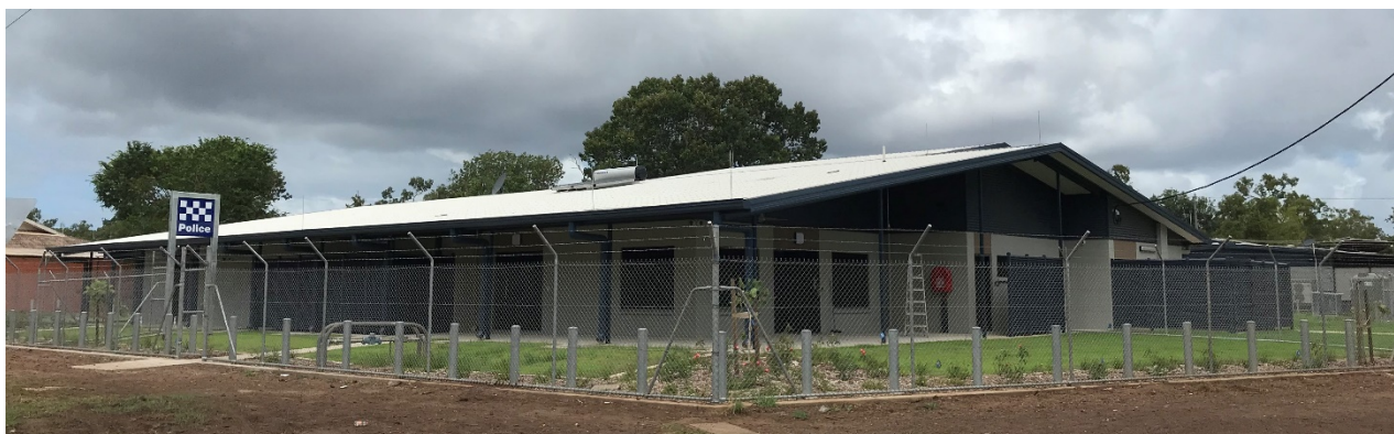
Construction photo: Angurugu - new permanent police post including multi-function area
