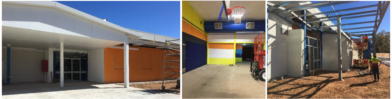
Construction photos: Centralian Middle School - gym upgrade
