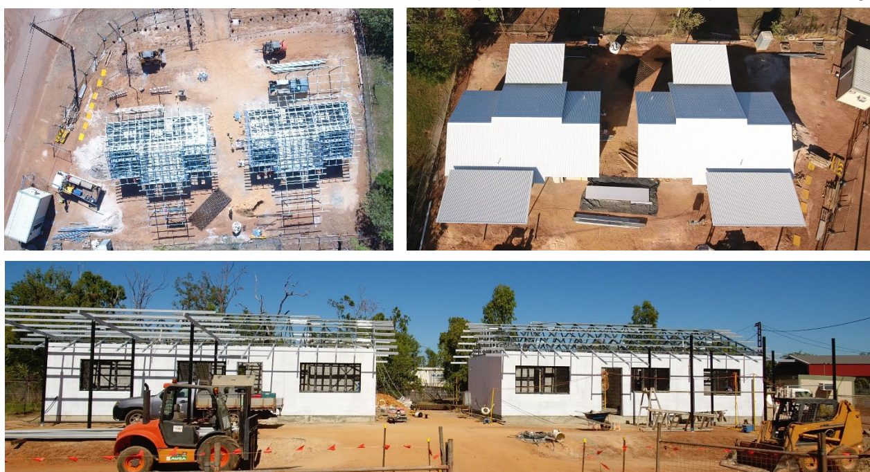
Construction photos: Beswick - construct 2 by 2 bedroom dwellings
