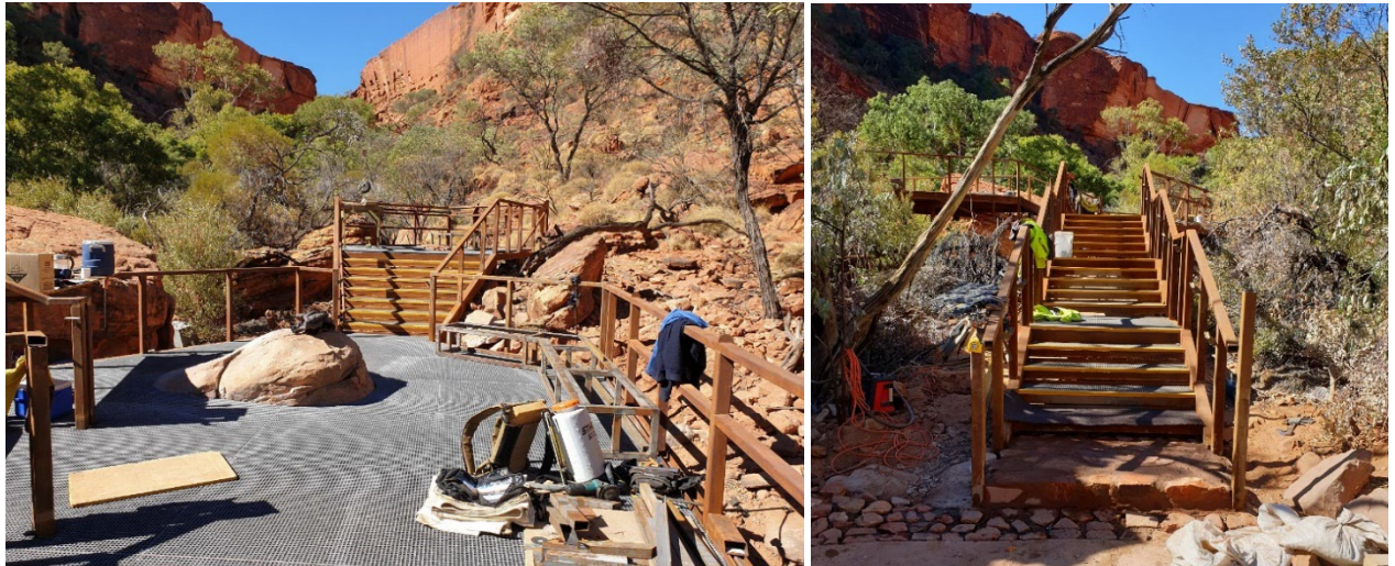
Construction photos: Watarrka National Park - Kings Creek viewing platform
