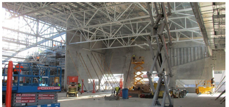
Construction photos: Darwin Middle School - new performing arts and multipurpose hall
