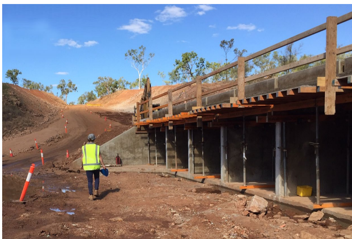
Construction photo: Wollogorang Road - Calvert River Crossing upgrade
