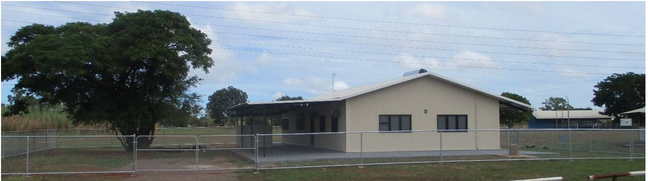
Construction photos: Town camps - urgent housing and infrastructure works
