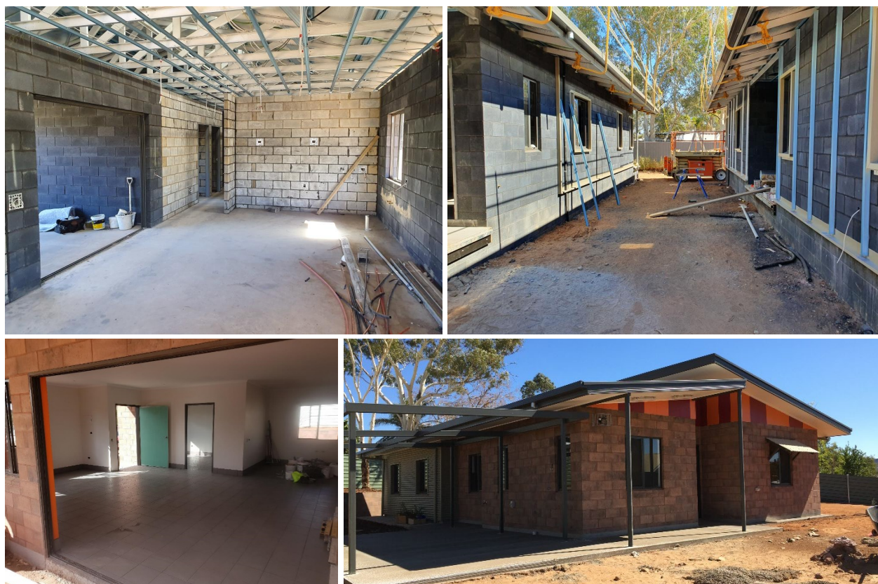
Alice Springs - design, documentation, demolition and construction of 14 new dwellings
