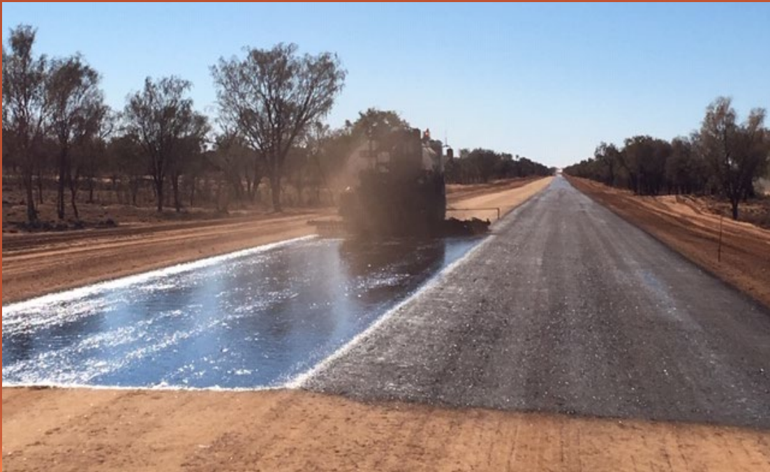
Plenty Highway - upgrade and seal - chainage 146.15 - 152.075 km
