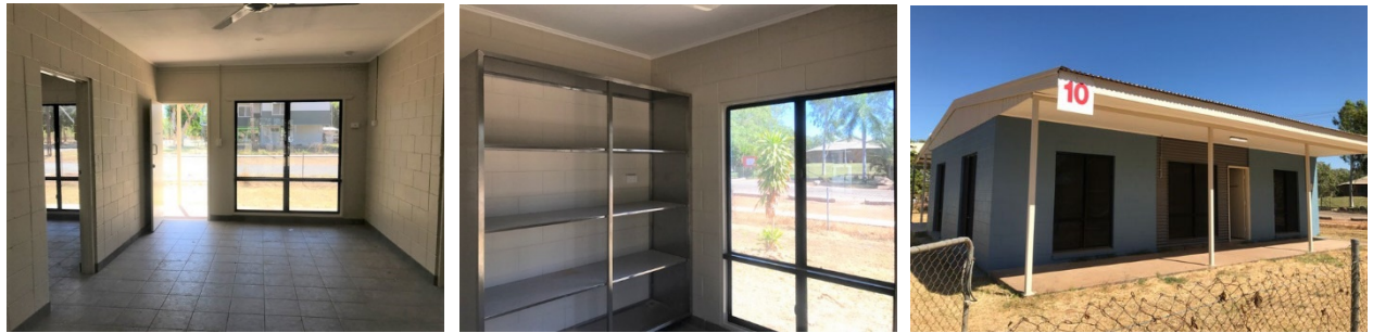
Construction photos: Town camps - urgent housing and infrastructure works
