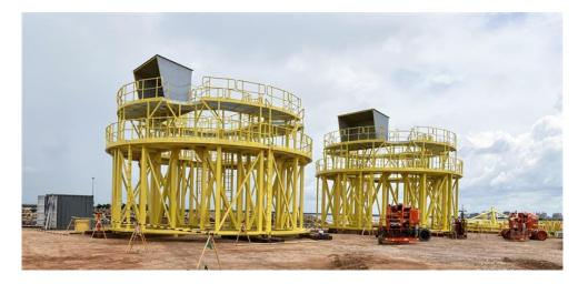
Construction of marine infrastructure for the Darwin Ship Lift Facility is set to start with the delivery of two caisson templates. These templates will be used to build the first seawalls for the project.
