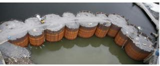
To connect the caissons, an arc template will be used. This template uses the sheet piles to form a hollow basin, which is filled with compacted rock (-75mm), to join the caissons to create a continuous seawall (*example picture above right*).
