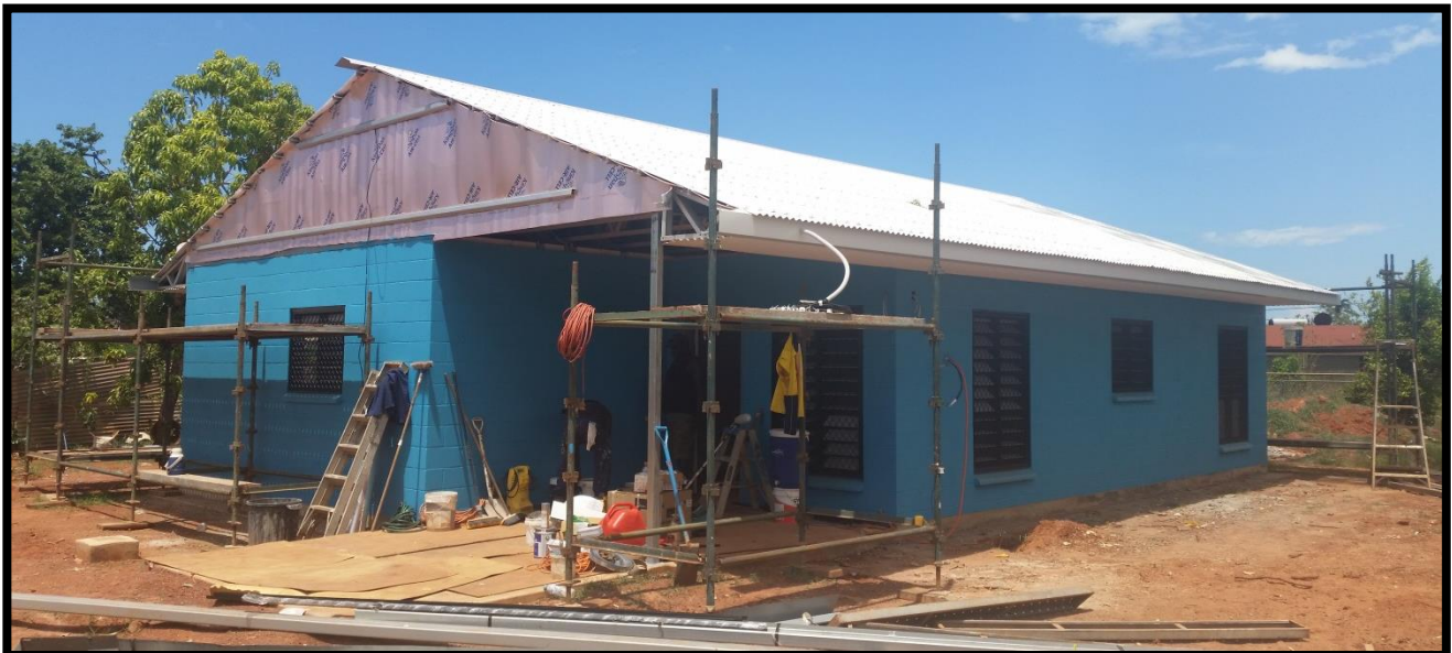
Photo: Ramingining, lot 122, demolish and replace 2 dwellings (cyclone recovery)
