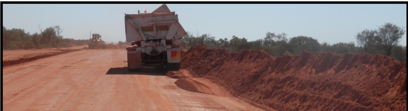
Photo: Tanami Road upgrade and seal
